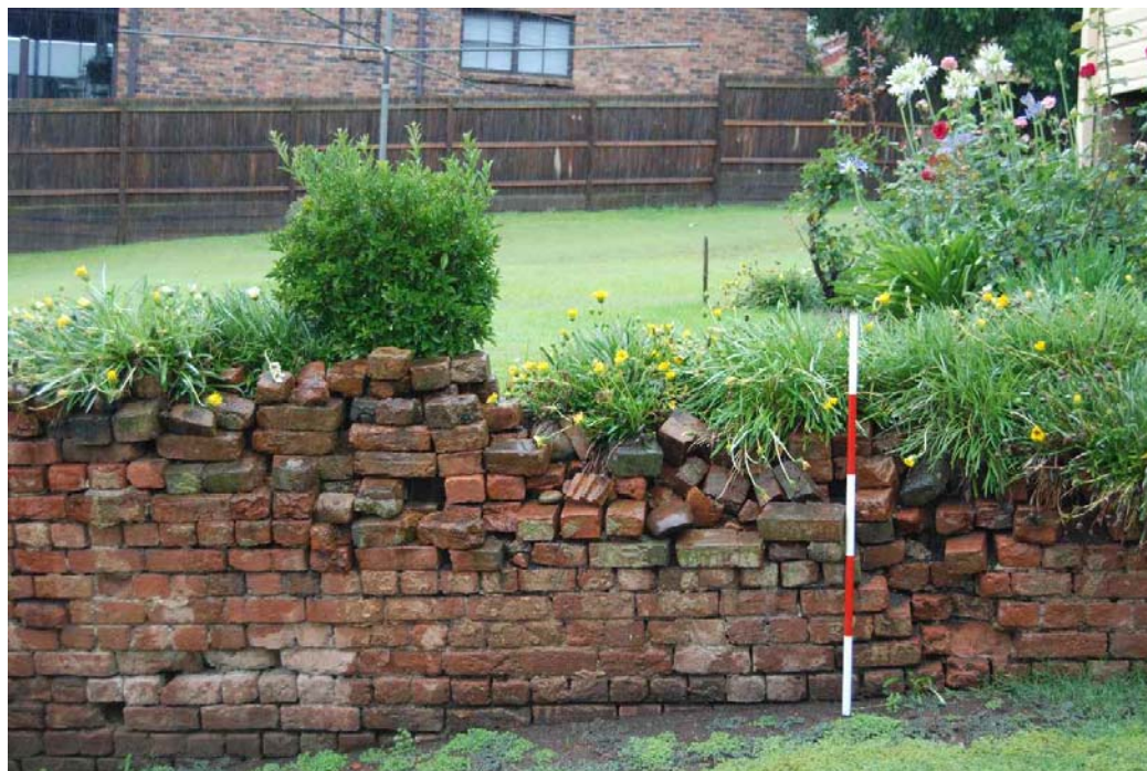
The sandstock brick retaining wall within the yard of 4 Bridge Street. View east.
