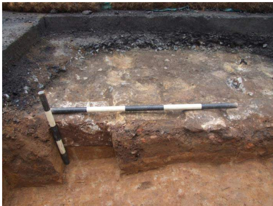
Figure 50: West facing view of SA 18 showing in section Telford type base layer [SA18-003] the mixed bedding material [SA18-004] beneath and the underlying natural mottled orange clay. A well-shaped block is seen at far left behind the vertical 50cm scale. The horizontal scale is 1m.
