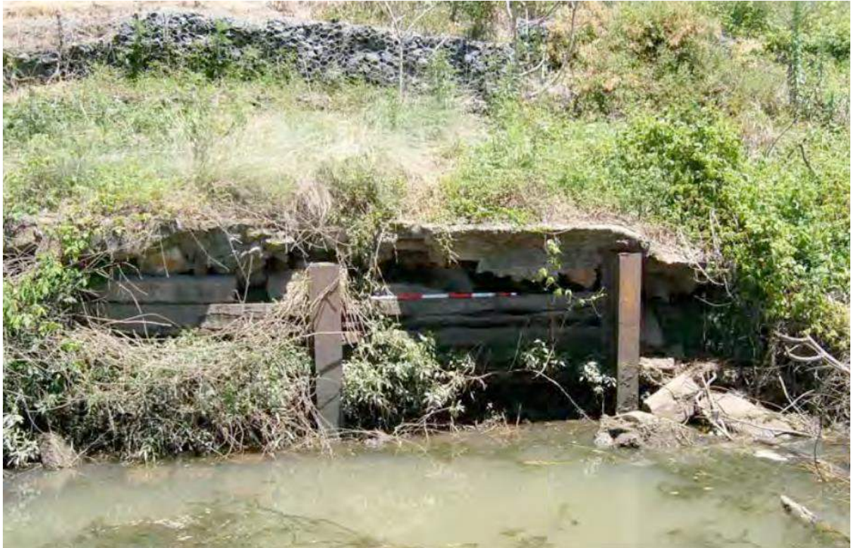
Figure 87: Remains of a retaining wall to the east of the above-water wharf remains. Recent gabion retaining extends across the waterfront, seen here in the background. (Source: Cosmos Archaeology).
