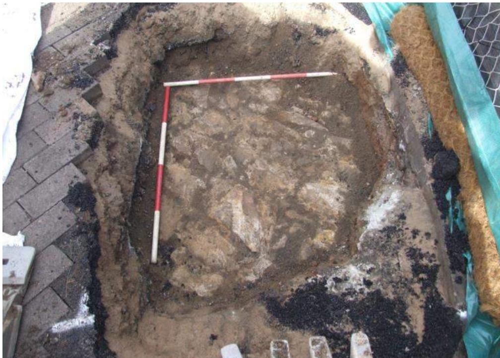
Figure 46: North-facing view of SA 16 showing the sandstone base [SA16-003] of the Telford road. The scales have 20cm sections.
