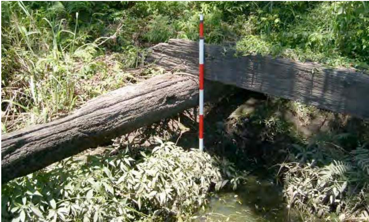
Figure 85: Remains of a deck beam and two walers of the 1820 wharf. (Source: Cosmos Archaeology).
