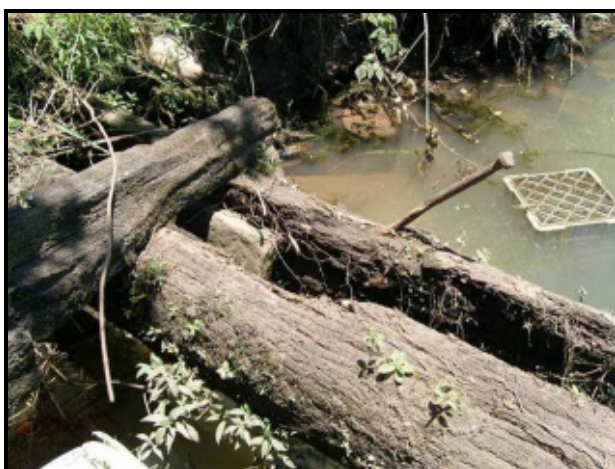
Figure 30: Fastening remains present on the two waler beams on the western side of the wharf remains (Photo Cosmos Archaeology).
