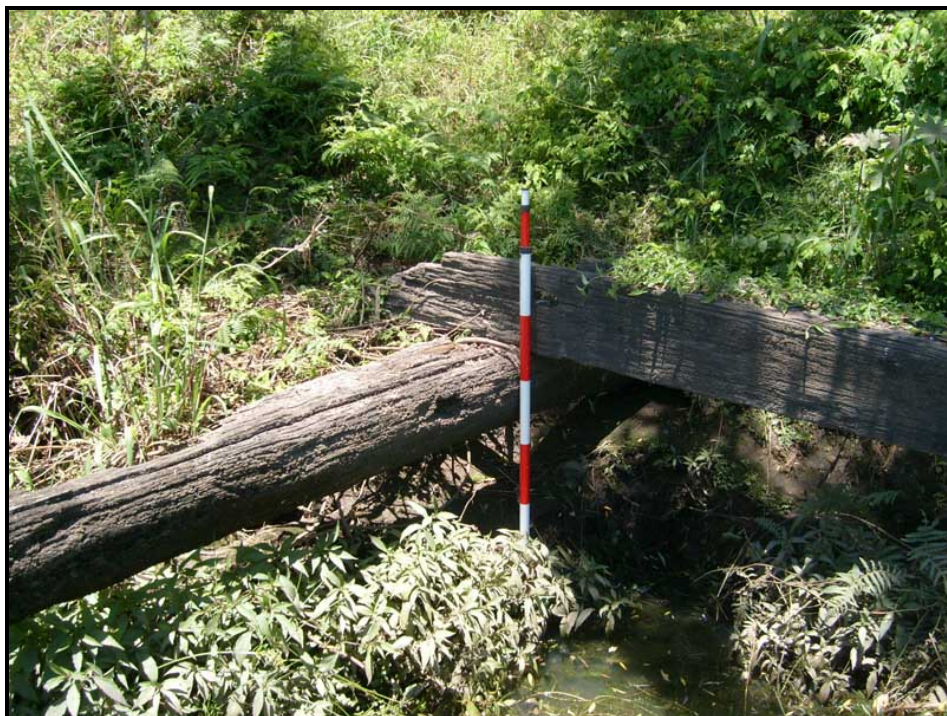
Figure 27: Remains of a deck beam resting on two walers. Scale in 200 mm increments (Photo Cosmos Archaeology).
