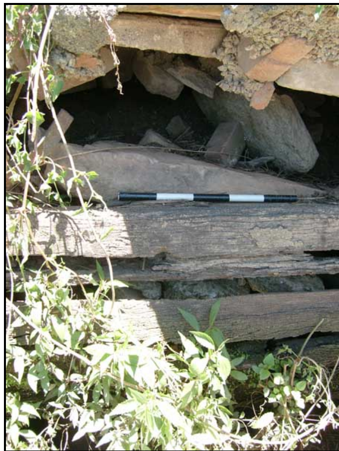
Figure 36: Example of the fill present behind the retaining wall. Scale in 200 mm increments (Photograph: Cosmos Archaeology).
