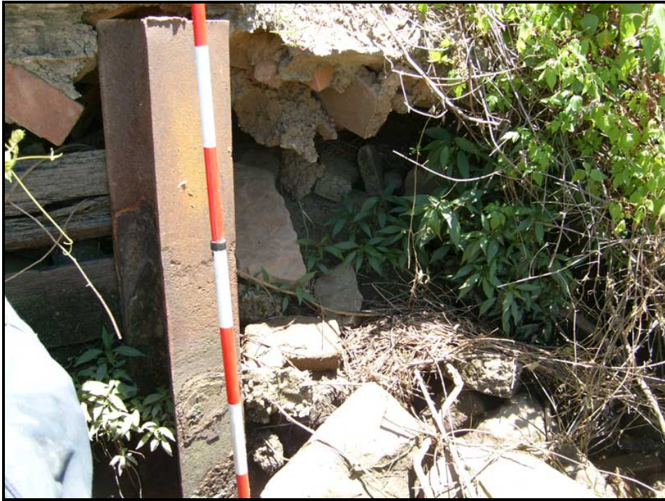
Figure 35: Iron girder that forms part of the retaining wall present on the riverbank. Scale in 200 mm increments (Photograph: Cosmos Archaeology).
