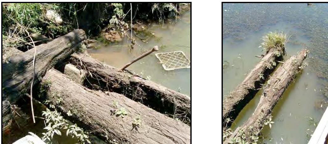
Figure 11: Fastening remains present on the two waler beams on the western side of the wharf remains (Photo Cosmos Archaeology).
