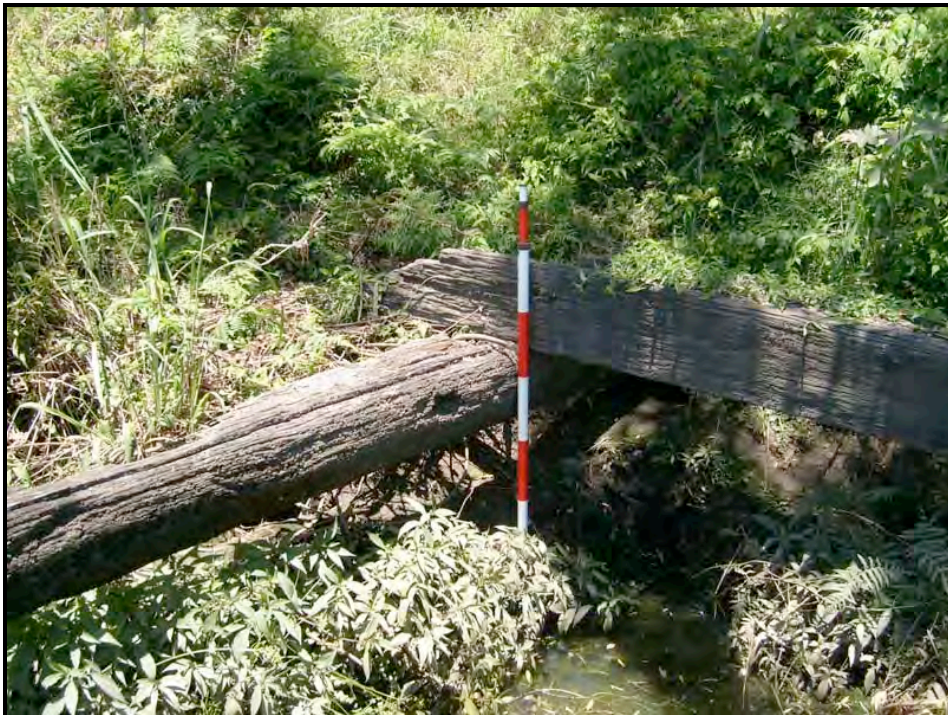
Figure 8: Remains of a deck beam resting on two walers (Photo: Cosmos Archaeology)
