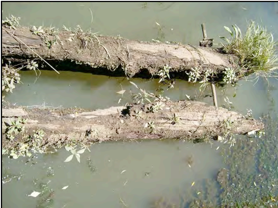
Figure 10: Remains of the two walers on the western side of the wharf remains (Photo Cosmos Archaeology)
