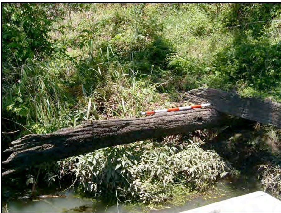
Figure 13: Remains of the singular waler on the eastern side of the wharf remains (Photo Cosmos Archaeology).
