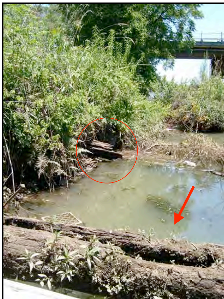
Figure 12: Recesses cut into the top of the walers (Red Arrow). Probable location of another deck beam. Note also the location of another waler in the centre of the photo (Red Circle) (Photo Cosmos Archaeology).
