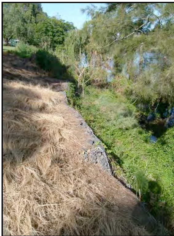
Figure 5: Gabion wall recently constructed above the location of the former wharf site (Photo: Cosmos Archaeology)
