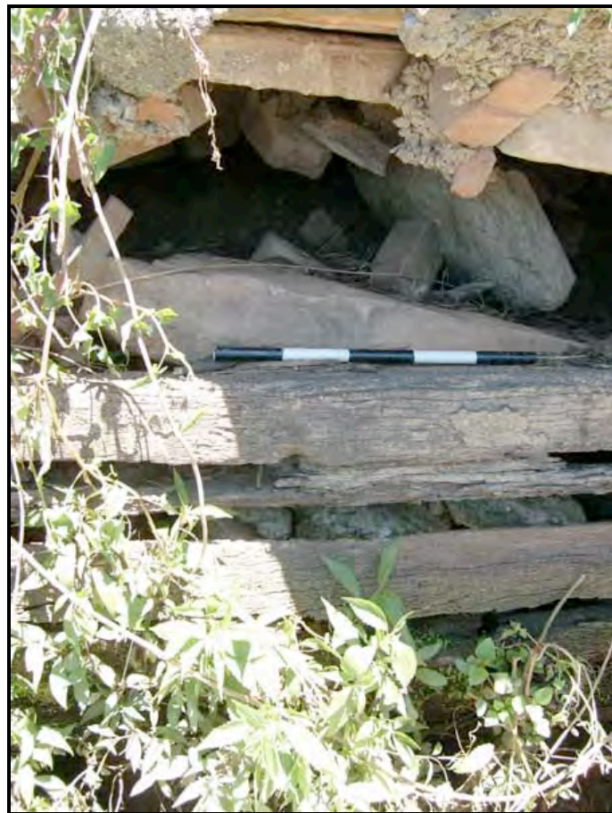
Figure 17: Example of the fill present behind the retaining wall (Photo Cosmos Archaeology).
