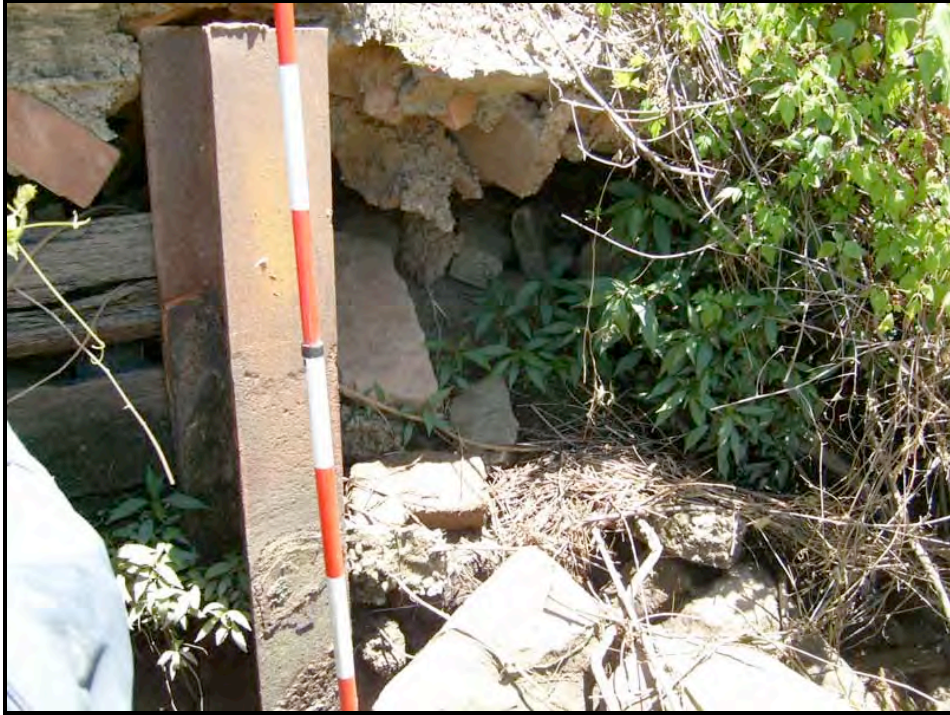
Figure 16: Iron Girder that forms part of the retaining wall present on the riverbank.
