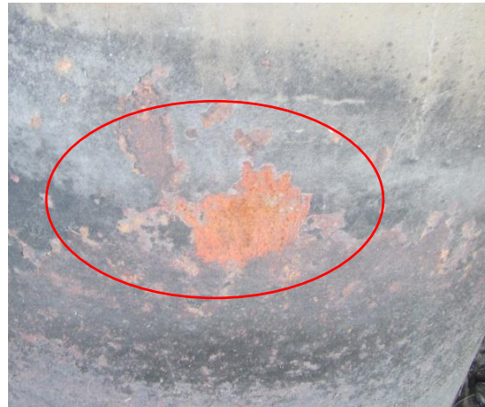
Figure 9: Localised corrosion on pier
