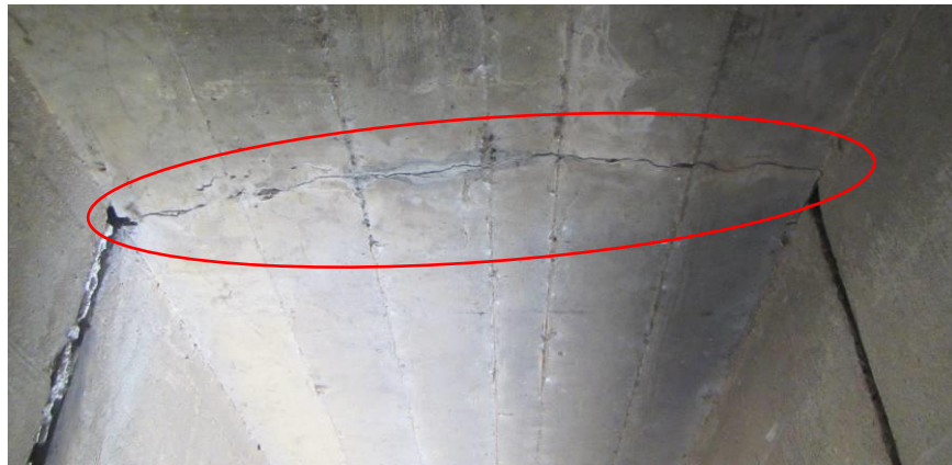
Figure 16: Crack in deck soffit between Span 1 and Span 2
