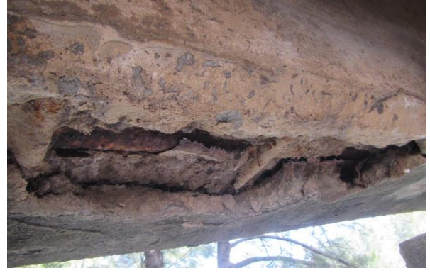
Figure 15: Spalling on Girder 1
