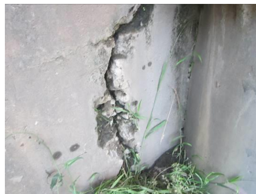
Figure 12: East wind wall vertical cracking, lower
