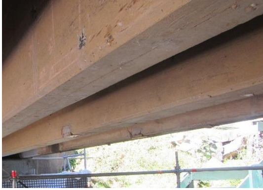
Figure 14: Typical interior girder condition (G2-G6)
