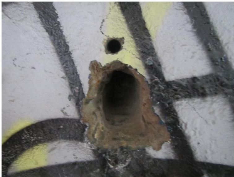
Photo 5 Abutment Wall Breakout B2
