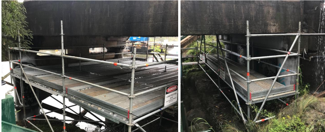
Figure 3 Scaffold setups for the investigation at the bridge
