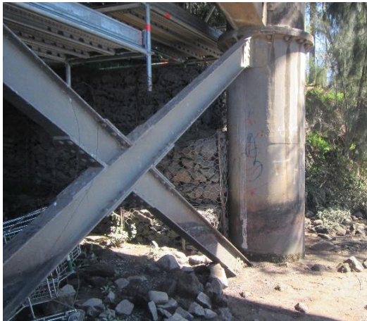
Figure 8: Span 1 cast iron piers and cross beams
