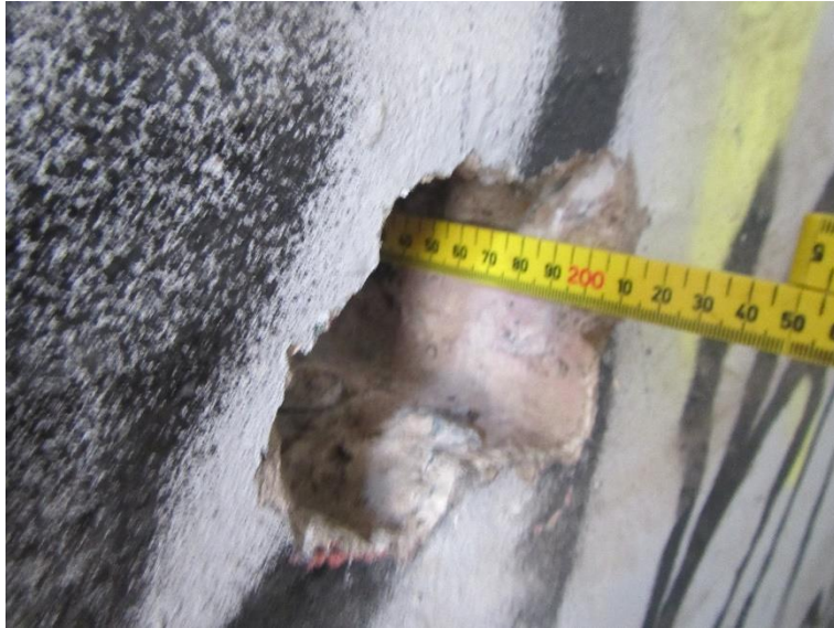
Photo 4 Abutment Wall Breakout B1
