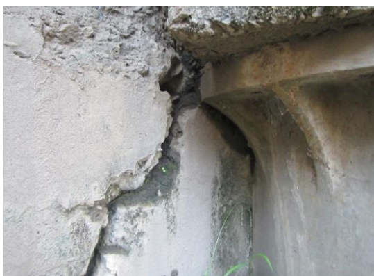
Figure 11: East wing wall vertical cracking, upper
