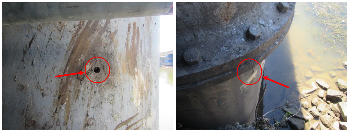
Figure 19: Pier 1 East Column core hole in the upper section (Left) and the lower section (Right) from the past investigation
