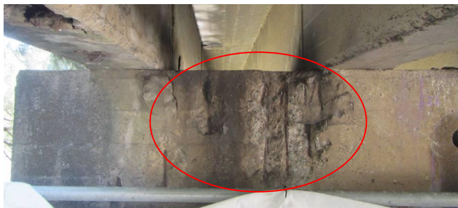
Figure 7: Area of spalling on Headstock 1 south face, west side
