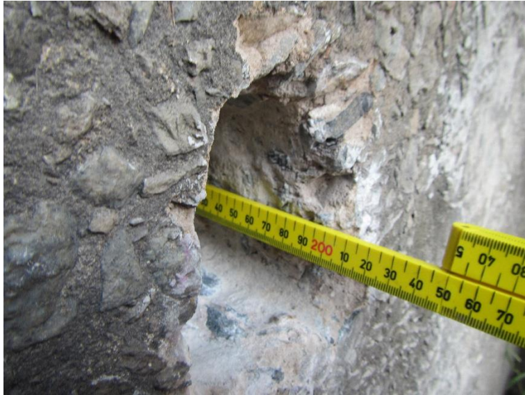
Photo 1 East side Wingwall Breakout B1
