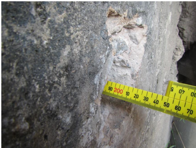
Photo 2 East side Wingwall Breakout B2
