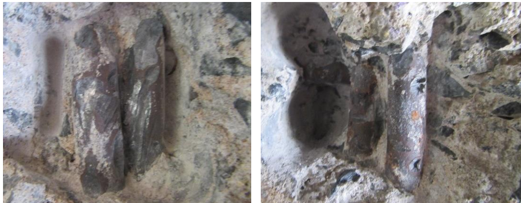
Figure 18: General condition of reinforcement in breakouts
