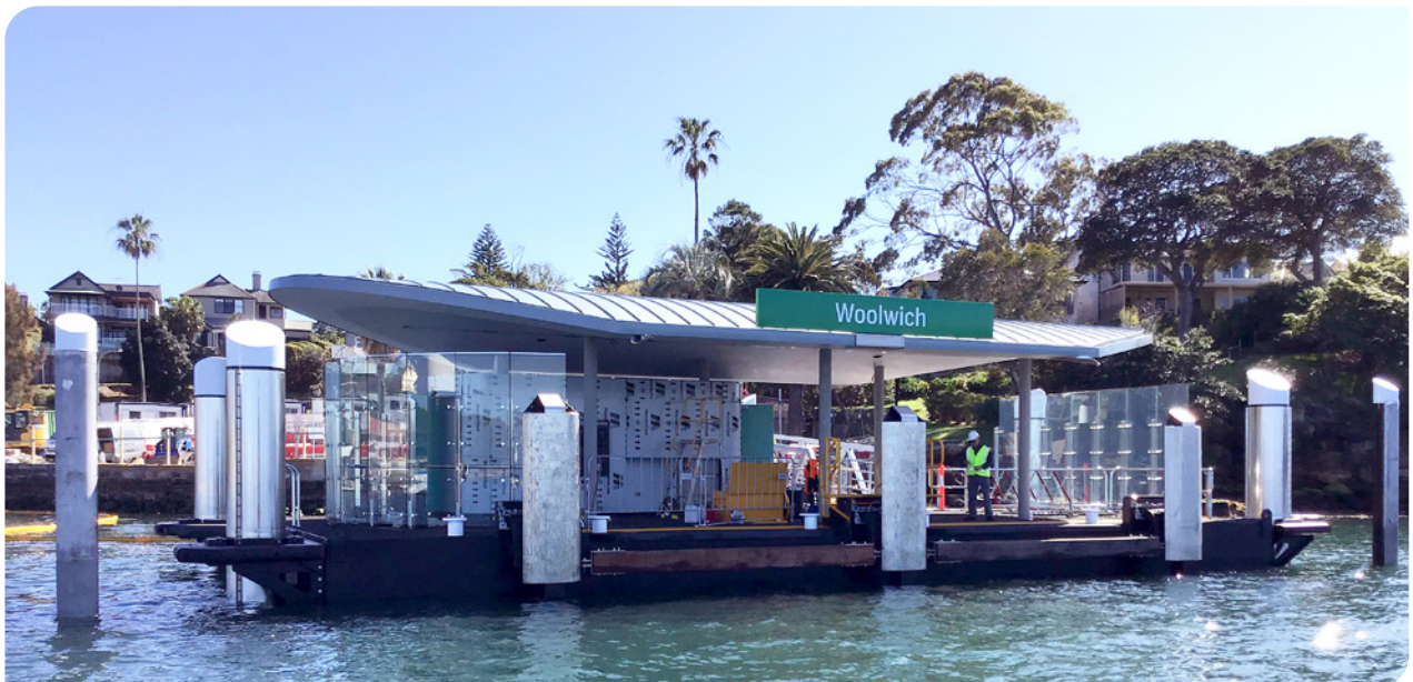
Woolwich Wharf construction nearing completion
