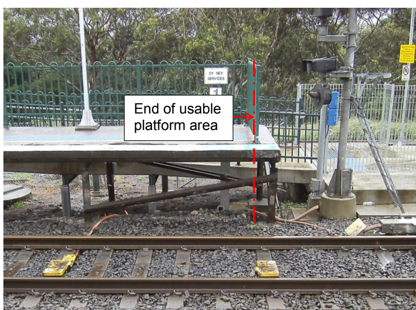
Figure 11: Measurement point for Edge of Platforms
