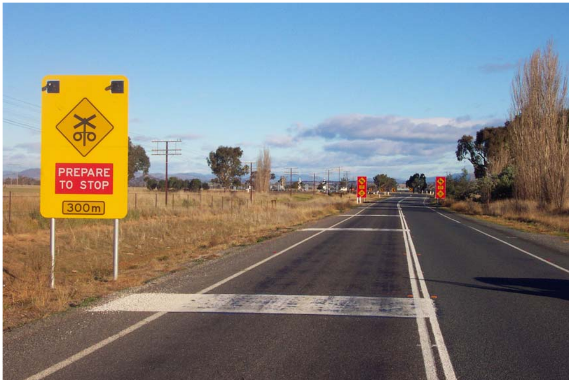
Advanced Warning Improvements - Olympic Highway (Bells Rd) Level Crossing - Gerogery
