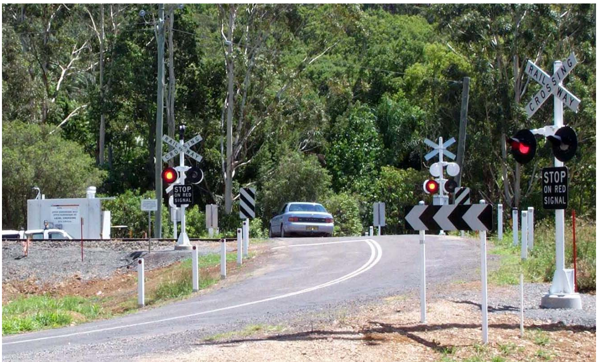
Upgrade to Type-F Active Protection - Upper Burringbar West (Upper Burringbar Road)
