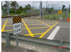
28 Minor upgrades were completed. Minor safety upgrades include the installation of high intensity lamp units, signage and road markings. Earthworks to improve motorists sighting of approaching trains are also carried out as part of minor safety upgrades.
