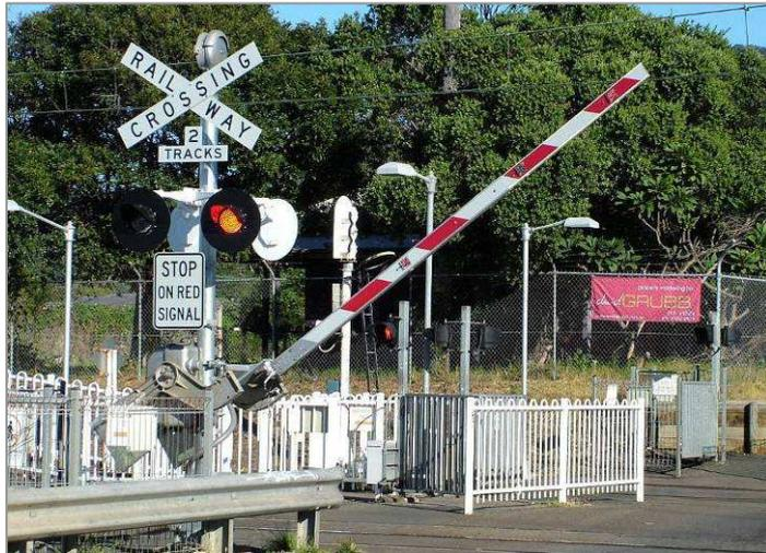
Commissioned on 7 May, 2006, the \$27,000 minor works upgrade at Bellambi (pictured) included new boom gates, provision of Safeflash, high intensity (LED) lights, width marker signage and removal of non frangible structures on the northern side of the rail line. New pedestrian lights were also installed.
