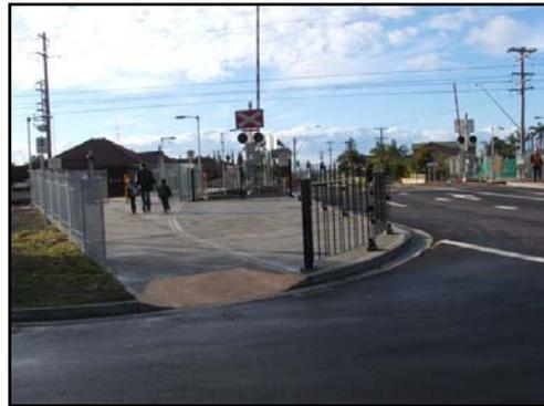
An existing pedestrian level crossing was renewed and a new pedestrian level crossing was installed to reduce pedestrians' and cyclists' need to use the road. Both pedestrian crossings are now compliant with disability access standards.
