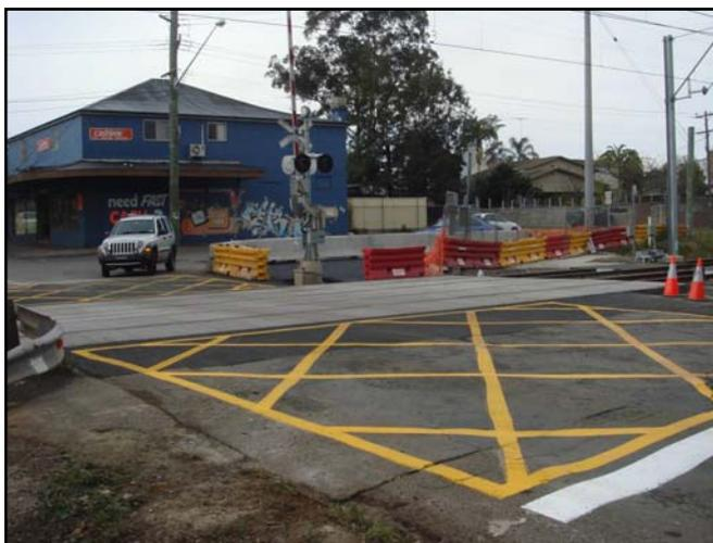
The upgrade of the level crossing at Garfield Road, Riverstone is being completed in stages and is expected to be commissioned in March 2010. Work planned for the site includes the interfacing of traffic lights and level crossing controls; minimisation of boom gate down-time; installation of a new pedestrian crossing; and improved street lighting and pavement markings.
