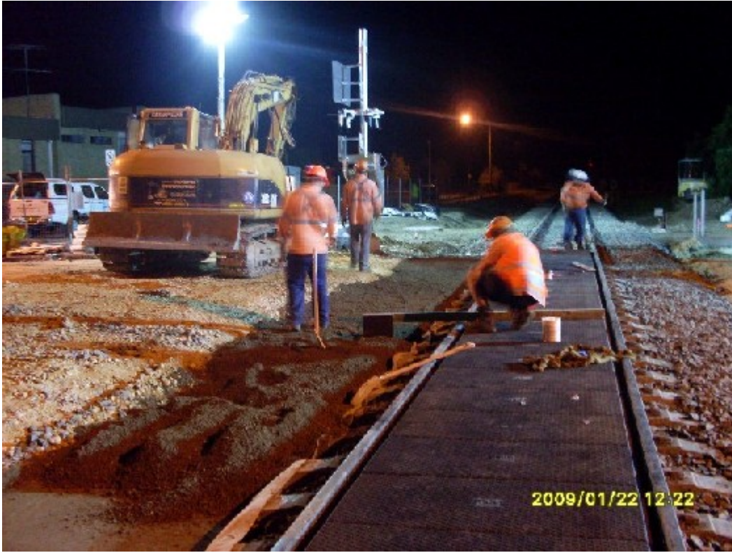
Figure 1: Night work construction of the Scone level crossing
