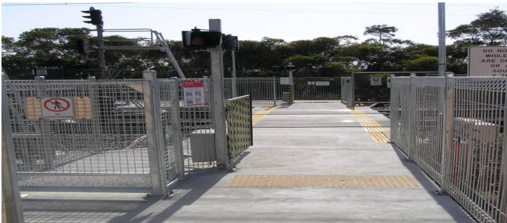
Figure 5: Cowan Station Northern Line
