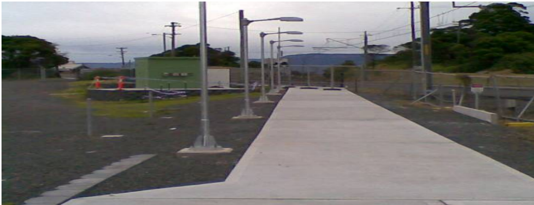
Figure 8: Unanderra Princes Hwy Pathway and Lighting (Illawarra Line)
