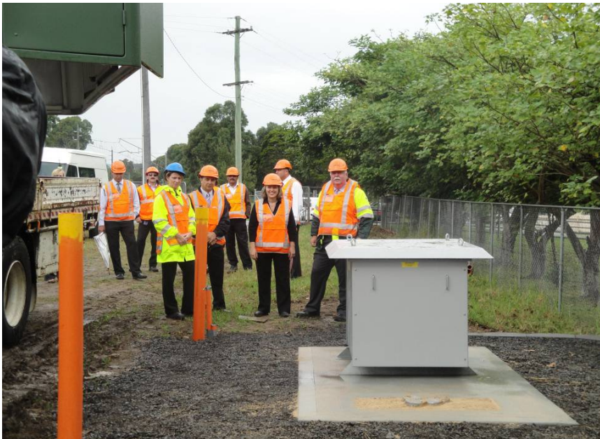
Figure 7: Installation of new power supply Avondale Rd Dapto (Illawarra Line)
