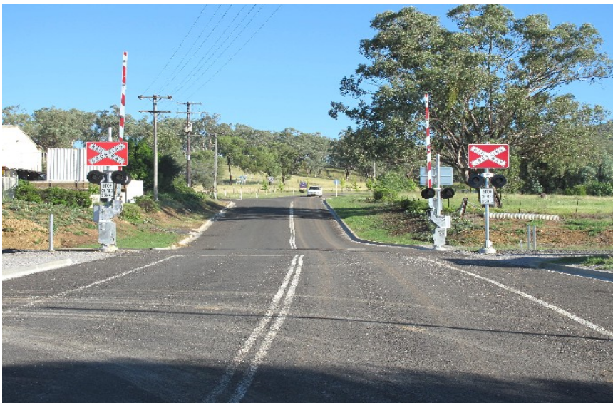
Figure 4: Level crossing at Nemingha – after, with active controls, boom gates, flashing lights and bells.
