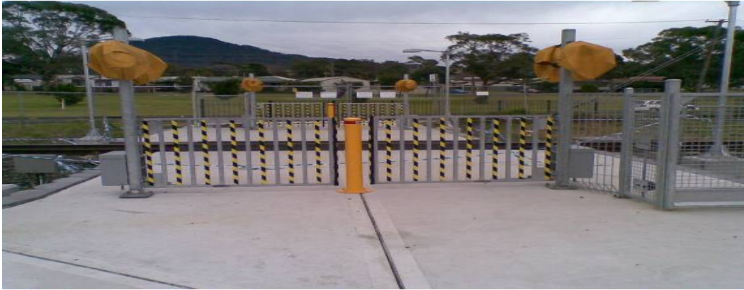
Figure 9: Unanderra Princes Hwy Swing gates (Illawarra Line)
