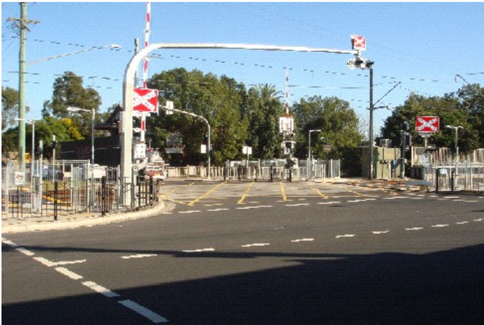
Figure 10: Riverstone Garfield Rd Metro West Line
