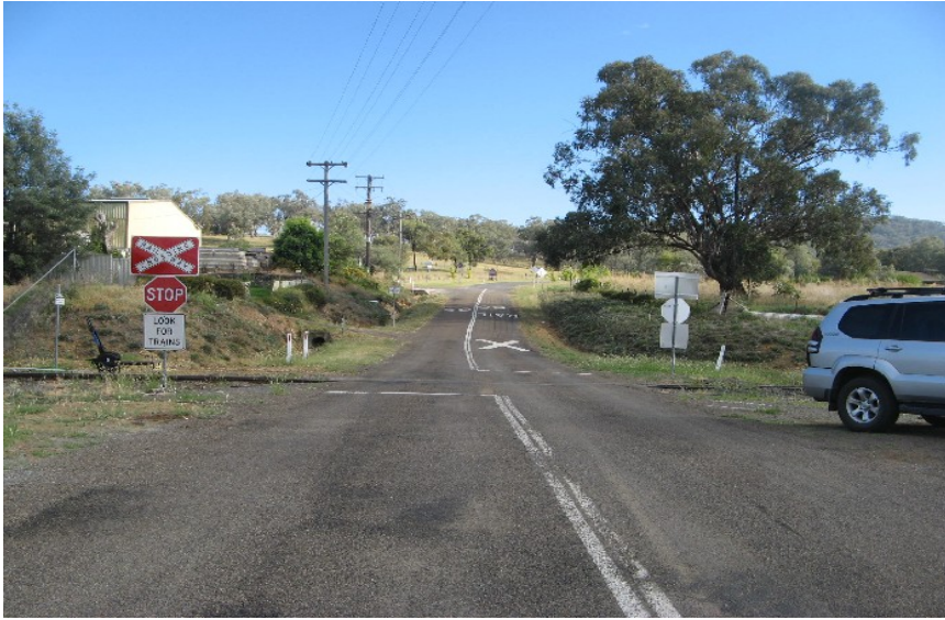
Figure 3: Level crossing at Nemingha – before, with passive “stop” control
