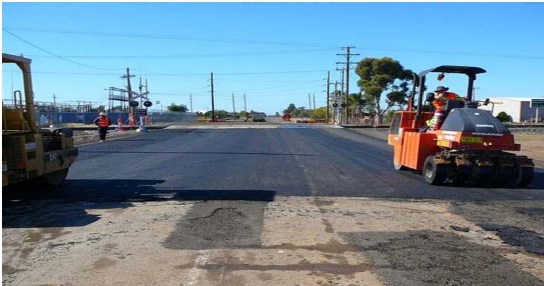
Figure 2: Construction of level crossing and road improvements at Bullus Drive, Moree
