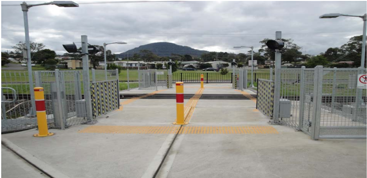
Figure 8: Unanderra Princes Hwy Swing gates (Illawarra Line).
