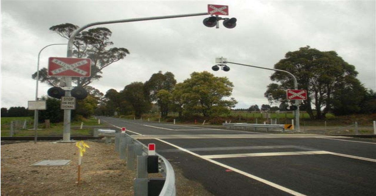
Figure 6: Sheep Wash Road, Calwalla level crossing.
