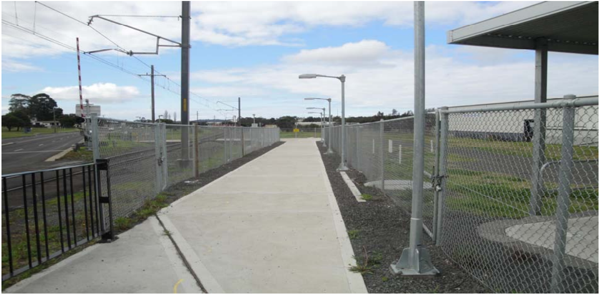
Figure 7: Unanderra Princes Hwy Pathway and Lighting (Illawarra Line).
