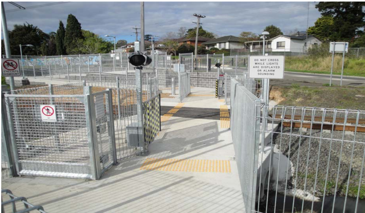
Figure 9: Avondale Road DDA compliant pedestrian and cyclist swing gate crossing.
