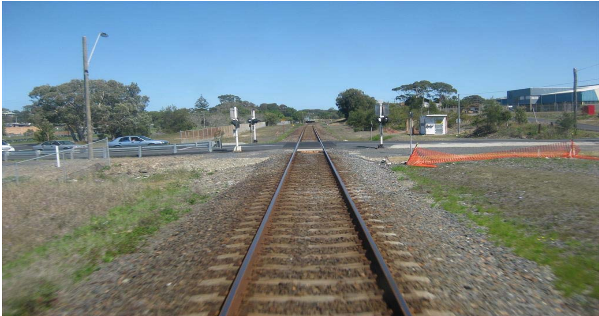
Figure 2: Sawtell level crossing under construction.
