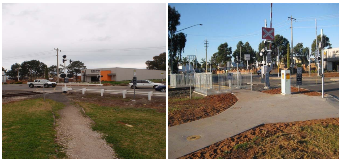
Figure 3: Before and after photos of the level crossing and road improvements at Blumer Ave, Griffith.
