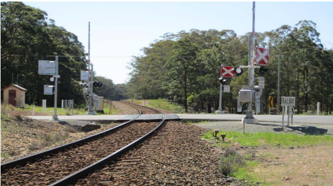
Figure 1: Kundle Kundle level crossing.
