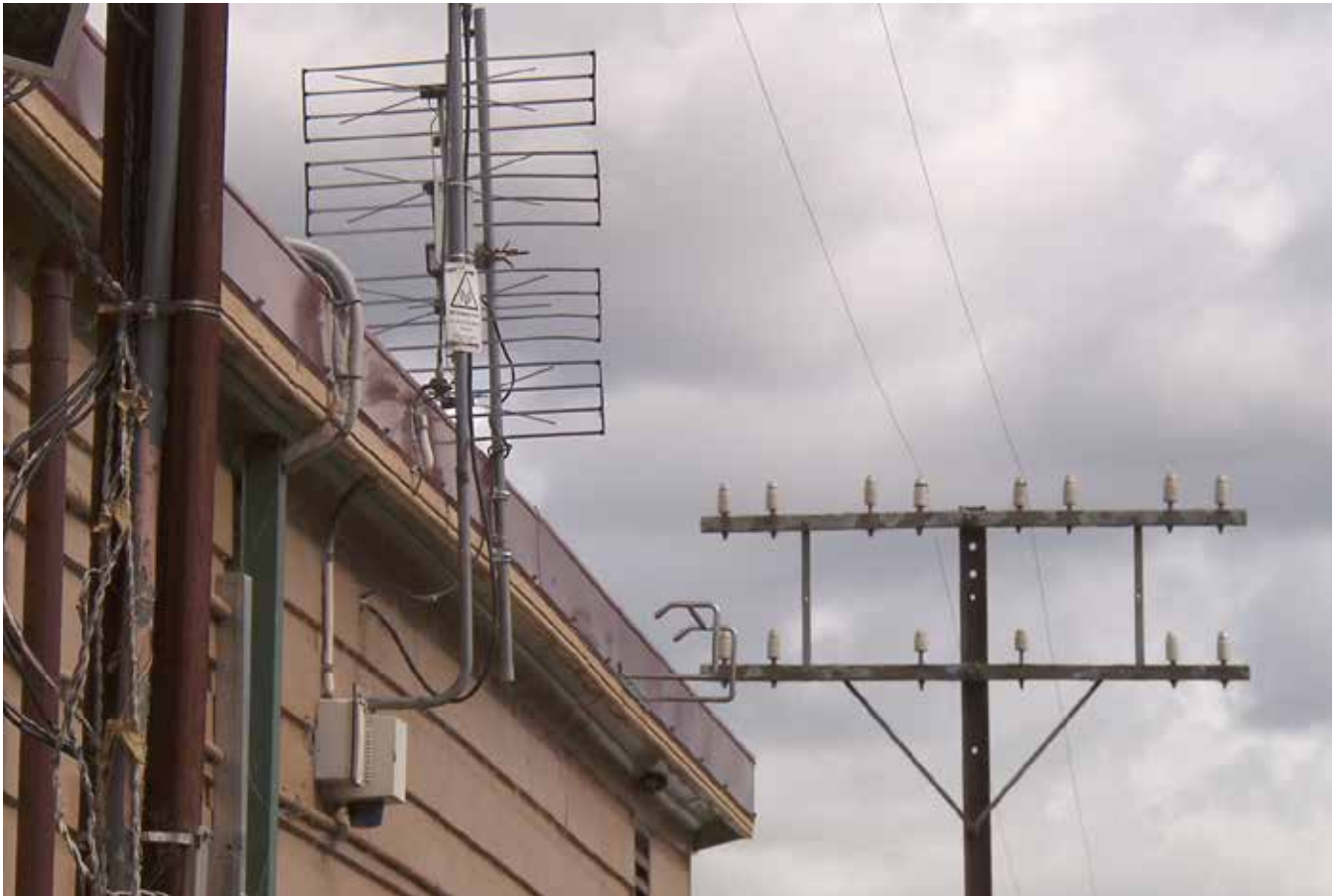
Copper line wire on upended rail tracks at Bomaderry Station. (Cinetel Productions)
