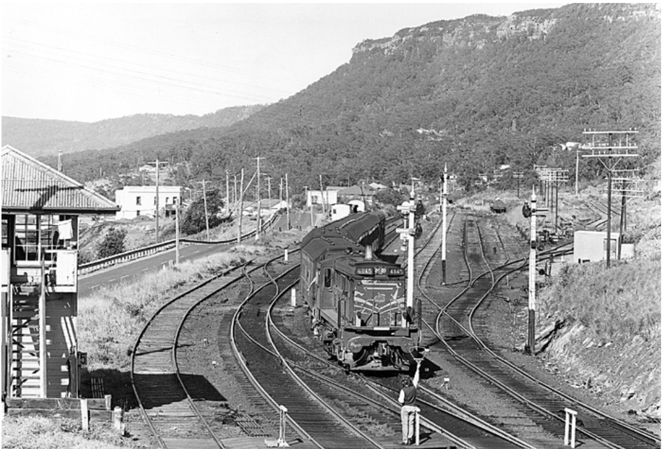
Guard holding up sling for exchange of staffs, Scarborough, 1981. (Courtesy of Australian Historical Railway Society, image no. 004501)
