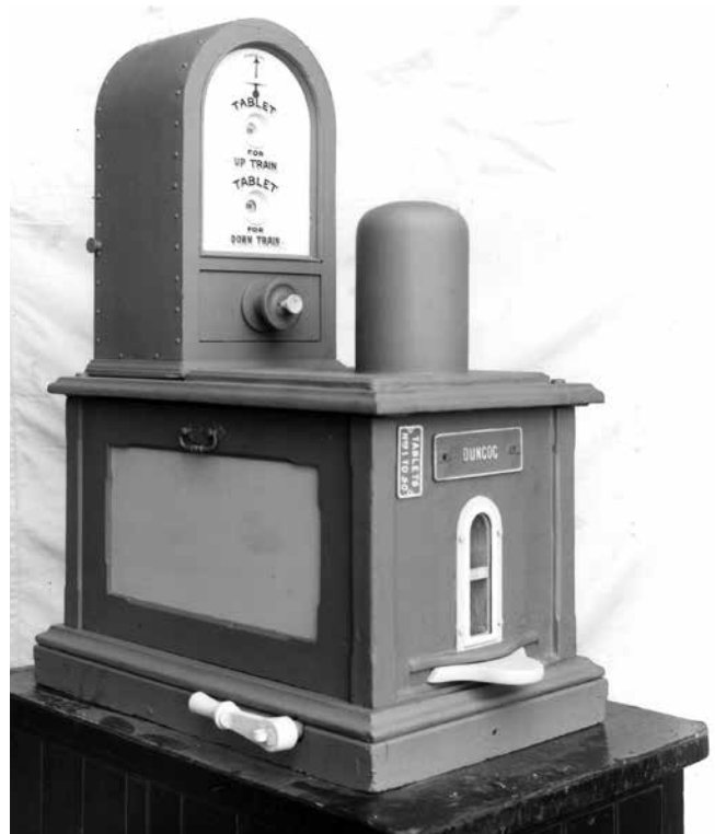
NSW Railways' Tyer's Tablet Instrument – most likely No. 3 pattern – the last of its type in-use in New South Wales. (Courtesy Robert Taaffe).
