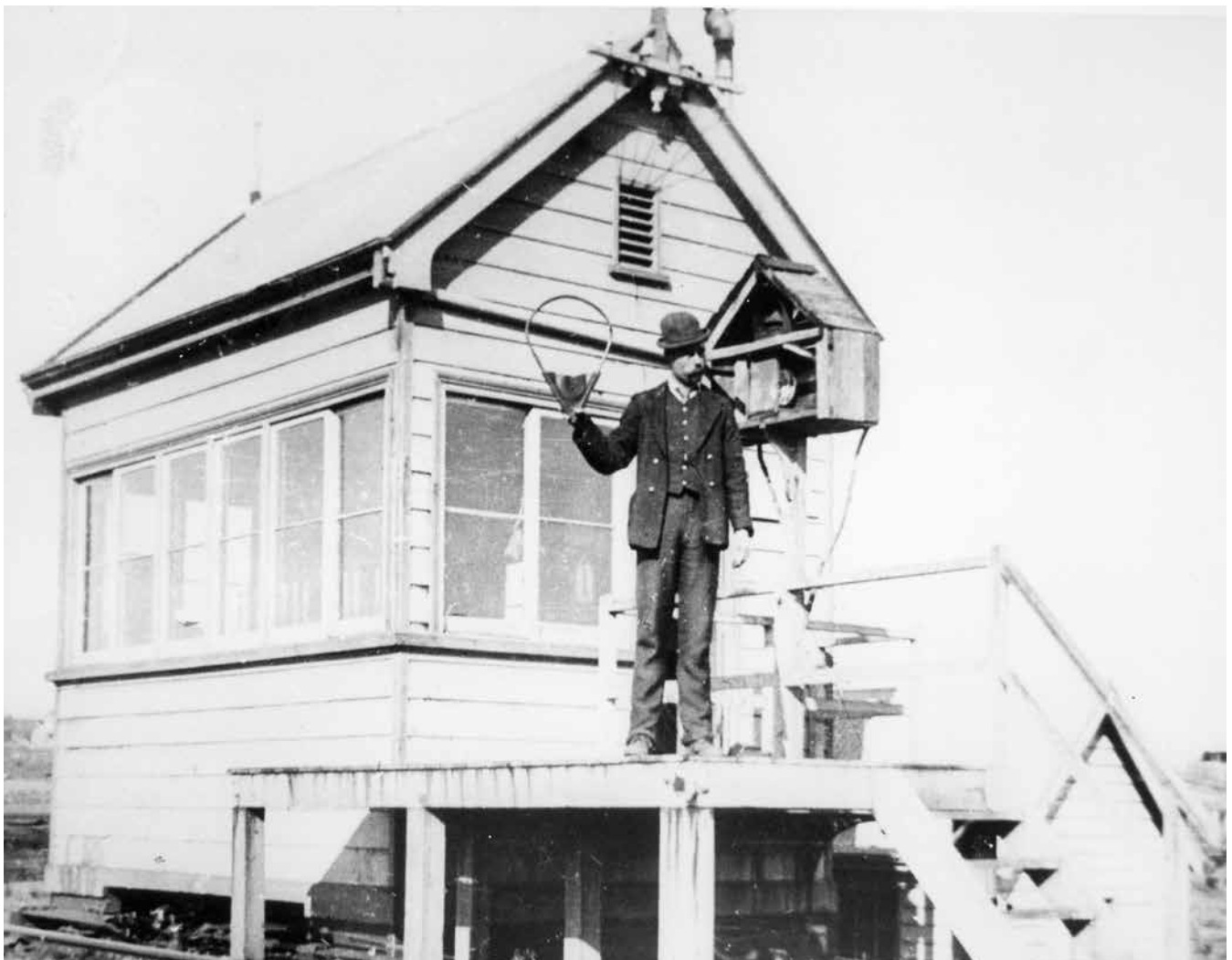
Train guard with tablet in sling, 1890s. Photo courtesy Australian Railway Historical Society, image no. 023611
