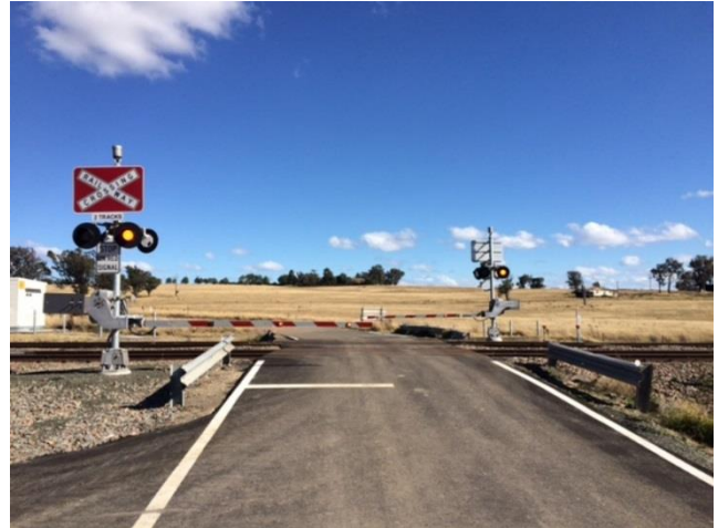
Middle Folbrook Road, Nundah (After)
