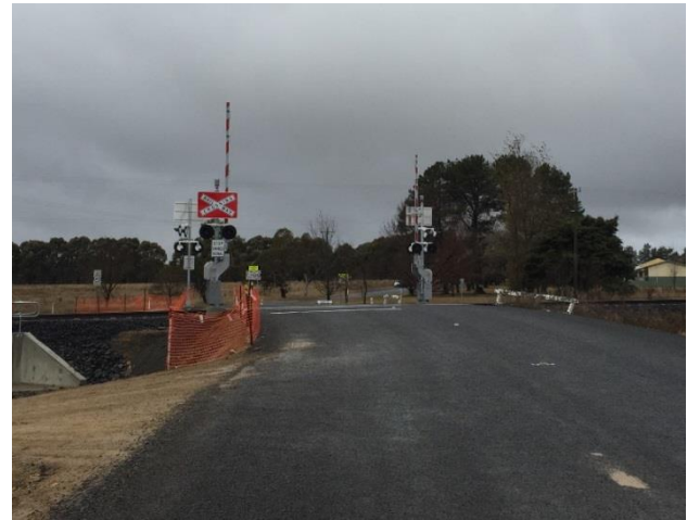
Clergate Lane, Clergate (After)
