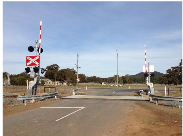
Yerong Street, The Rock (After)
