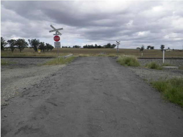
Middle Folbrook Road, Nundah (Before)
