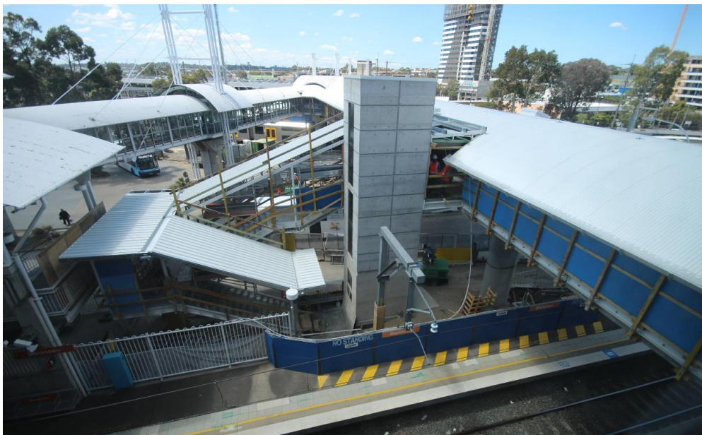
Construction work in progress for the new footbridge – November 2017
