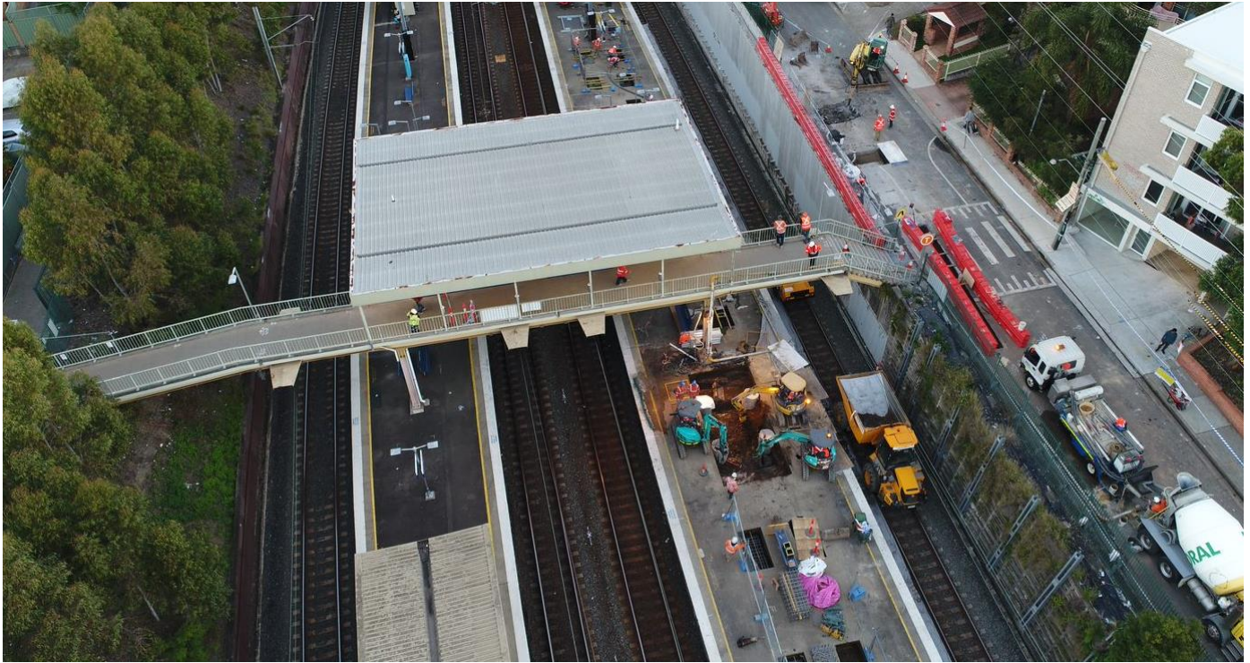
July 2017- Excavation commencing for underground works in preparation for lift shaft.
