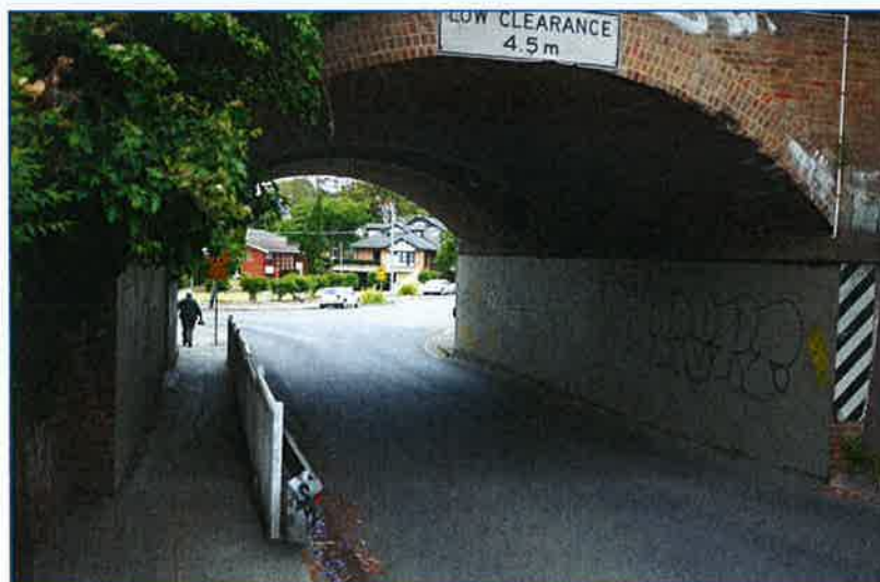
Figure 13: River Road underpass, eastern side.
