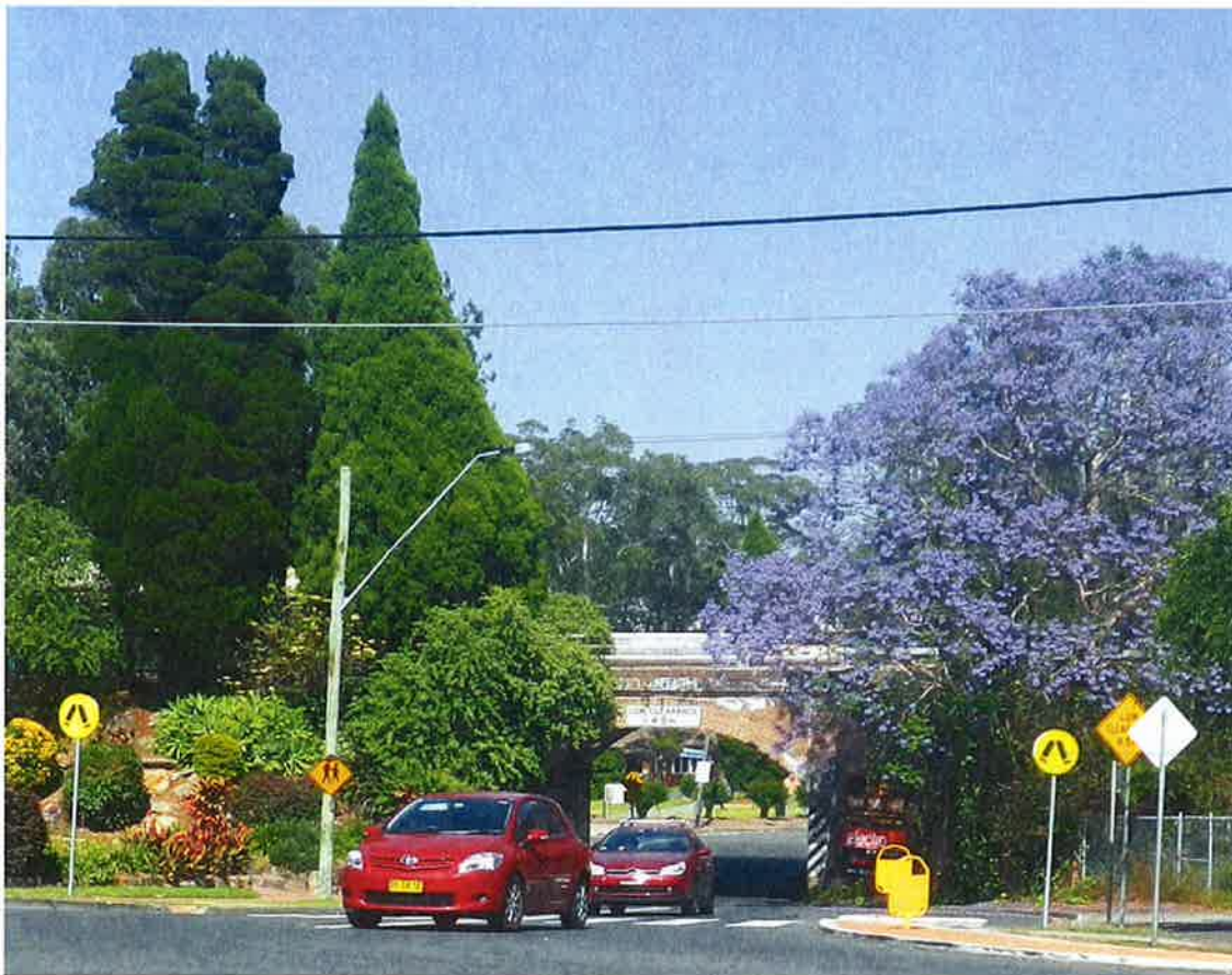
Figure 2: River Road Underpass view from the east
