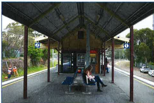
Figure 14: Northern end of station building.
