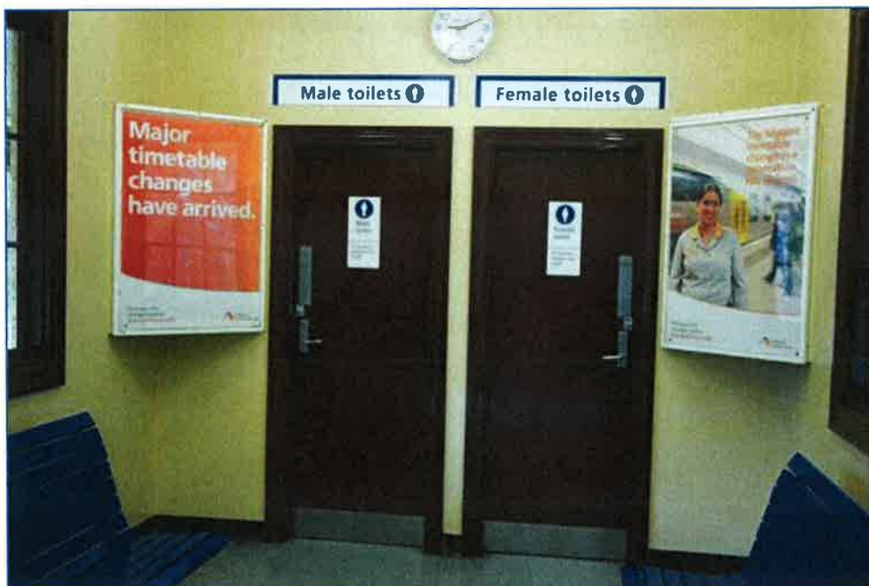
Figure 33: Existing toilet access.
