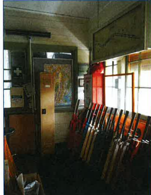
Figure 17: Signal room (facing north-east) including signalling levers and panel. Artefact Heritage 2012
