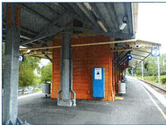
Figure 15: Southern end of station building.
