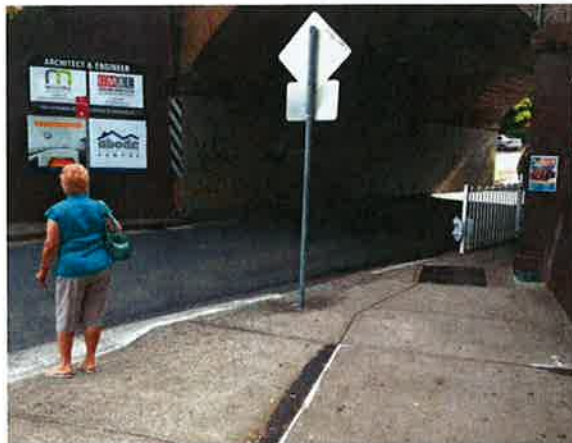
Crossing point considered unsafe (as per Road Safety Audit)
