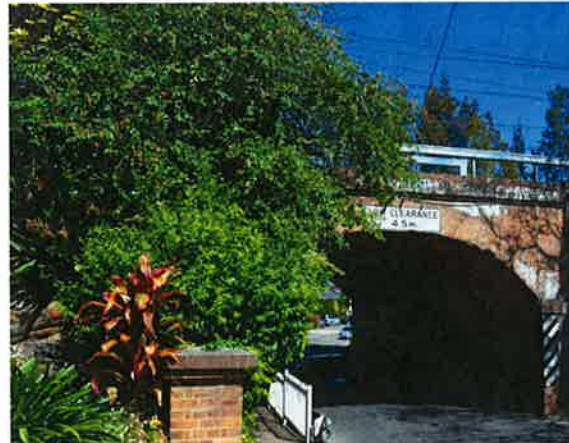
River Road underpass
