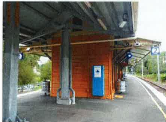
Looking north to the southern end of the platform building.
