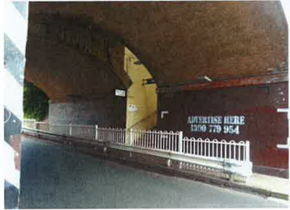
Narrow footpath at the entrance to the station
