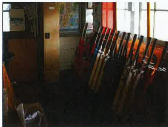
The lever room at the northern end of the platform building
