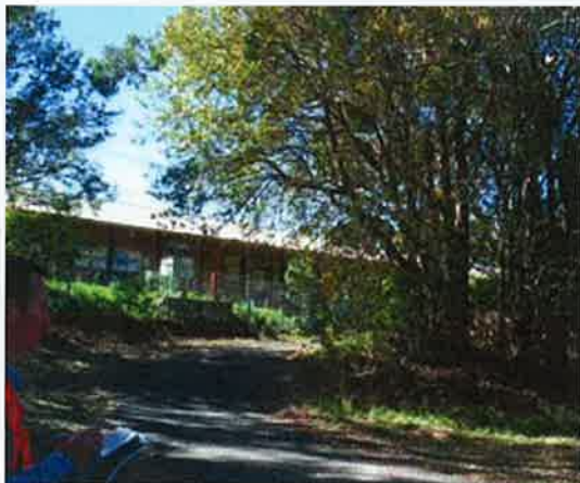
Access to RailCorp corridor on western side.
