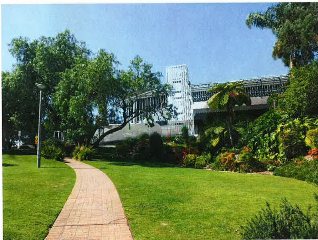
Figure 25: View from Douglas Cross Gardens (looking south), indicating proposed new works (Viewpoint 7)
