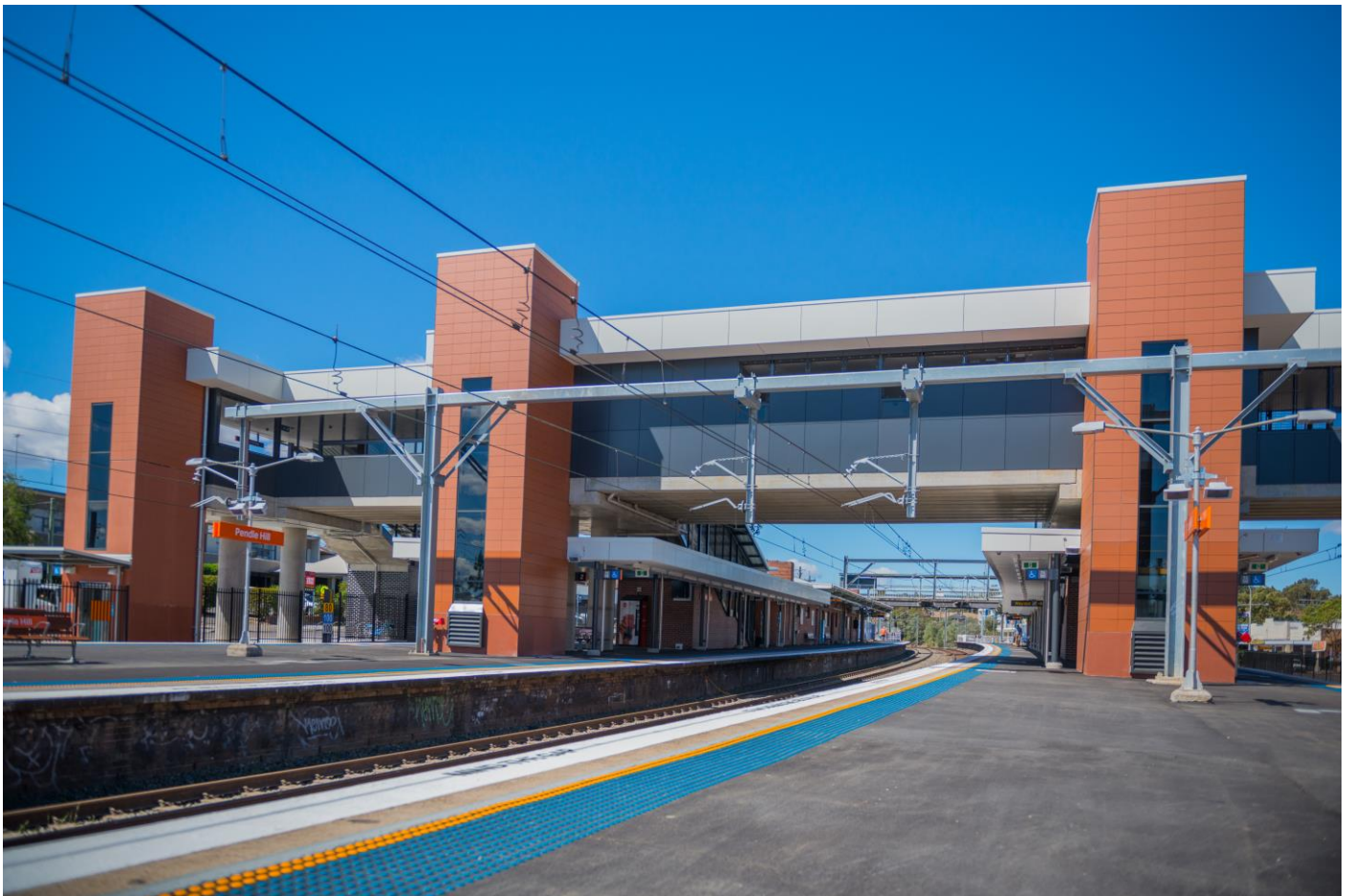
Pendle Hill Station after the station upgrade – September 2017
