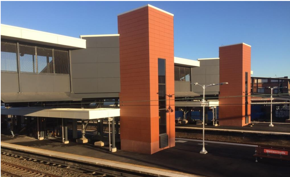
View of the new footbridge and lifts from Wentworth Avenue (August 2017)
