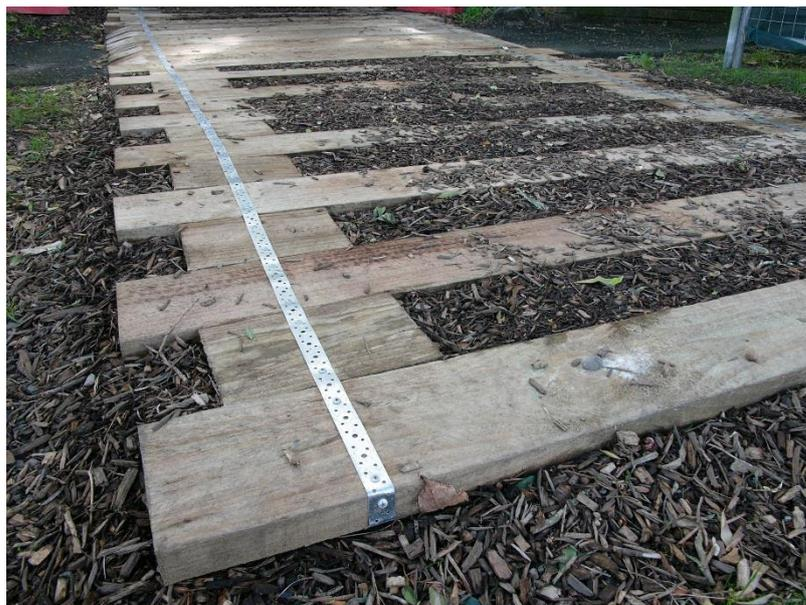
**Figure 7** – Showing typical detail for rumble boards.
