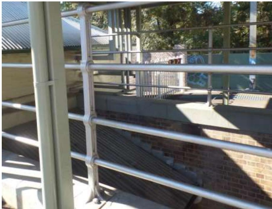
Figure 38. View into the stair ramp between subway and platform, showing the skillion roof to be removed and the location of the new concrete slab over the void to link both sides of the platform at this end.
