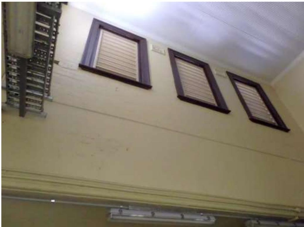
Figure 16. Interior of the pavilion, east side showing the louvres that now fill these openings
