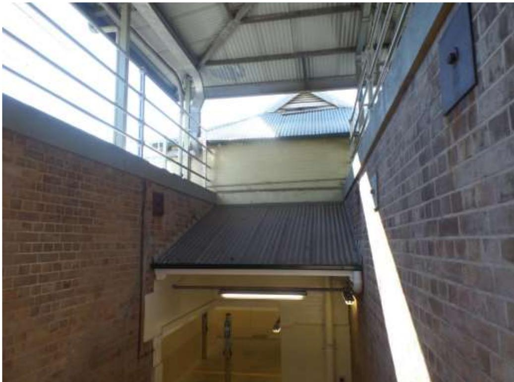
Figure 18. Platform stairs, showing the entry to the subway, the skillion rain shelter and the pavilion at the rear.
