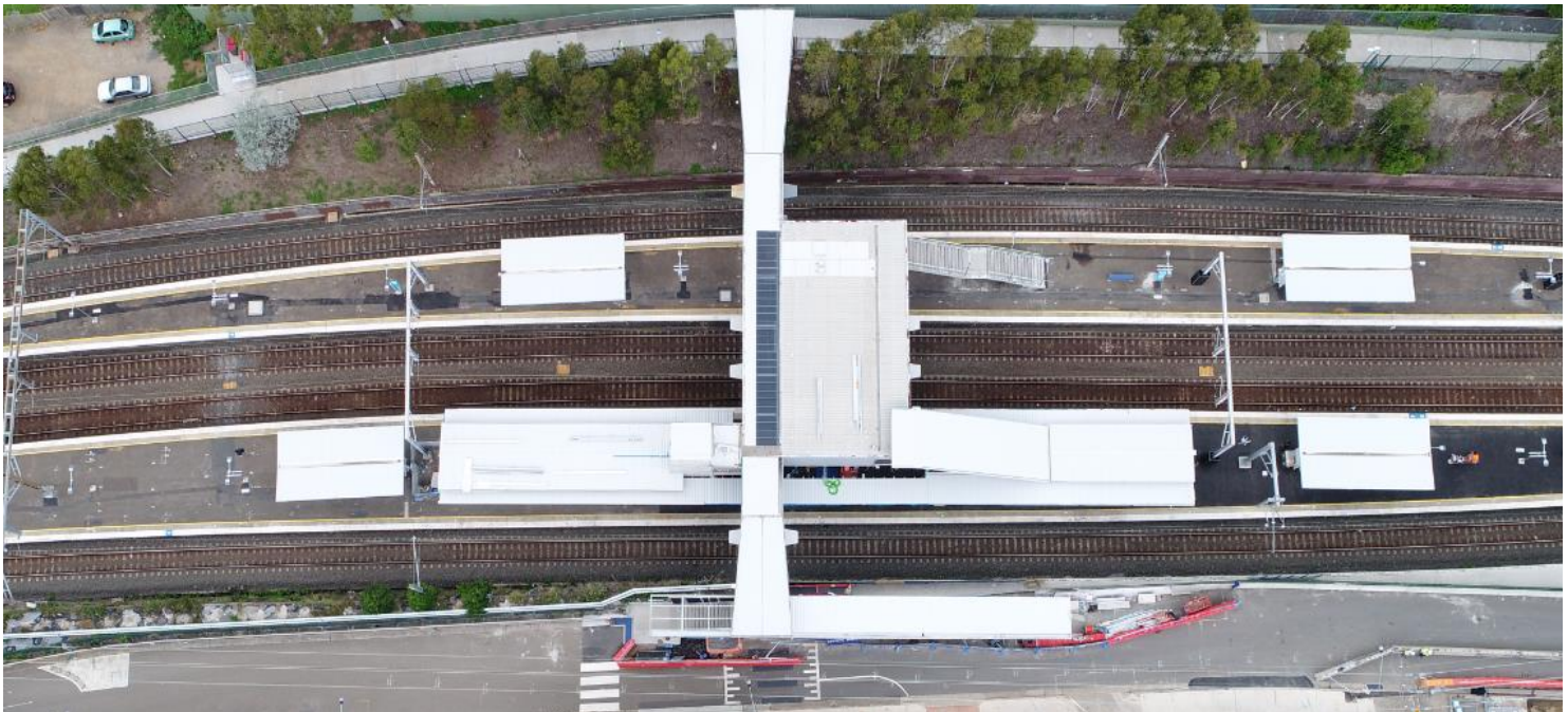
Aerial view of construction on Harris Park Station Upgrade
