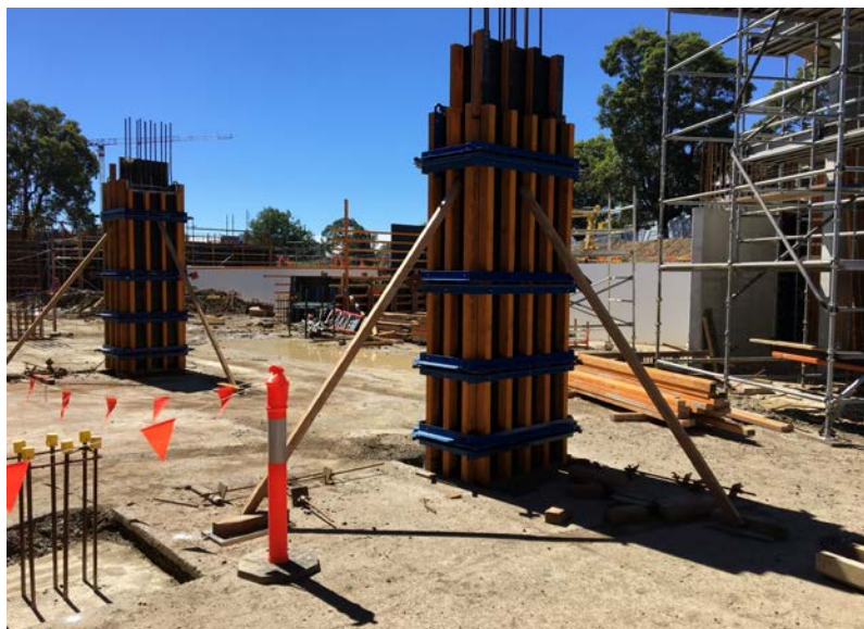
March 2018 – Columns poured at southern end of the Terminal Place site
