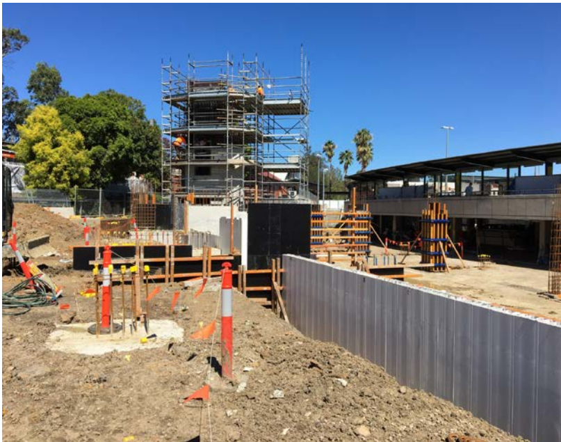
March 2018 – Lift pit formwork at the Terminal Place site.
