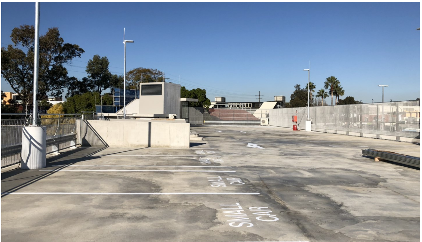
Construction of the top floor of the Merrylands Multi-Storey Car Park
