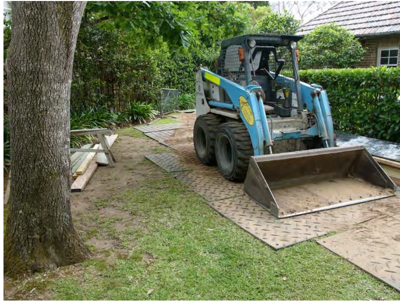
Figure 6 – Showing typical detail for truck mats.
