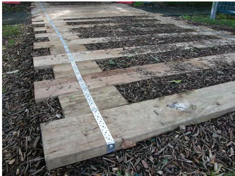
Figure 7 – Showing typical detail for rumble boards.
