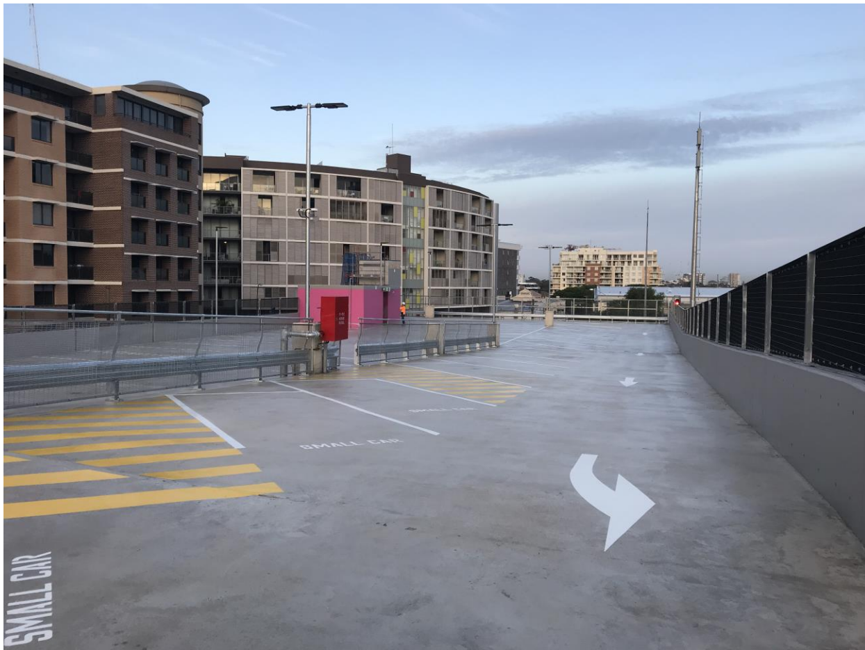
View from the roof of Ashfield Commuter Car Park – February 2018
