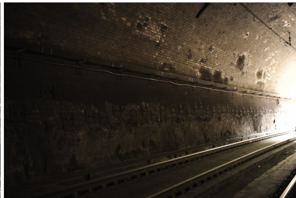
Figure 108: up track tunnel lining showing existing notching and rock bolts
