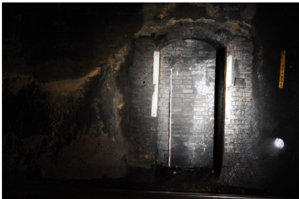
Figure 63: Brick arched and lined 'recess' in tunnel wall
