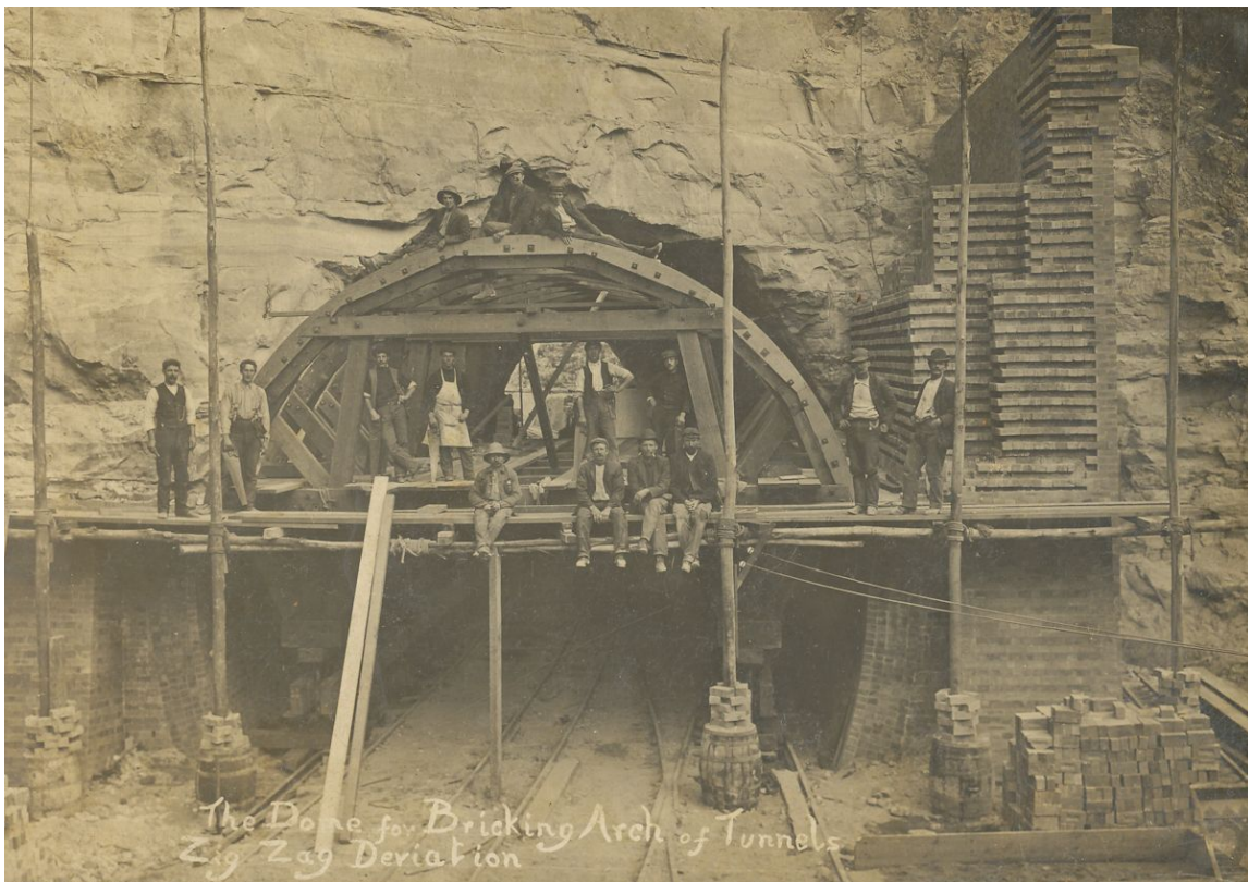
Figure 9: Workers during construction of the Great Zig Zag Railway deviation tunnels showing building of portal (Source: Lithgow Library Learning Centre)
