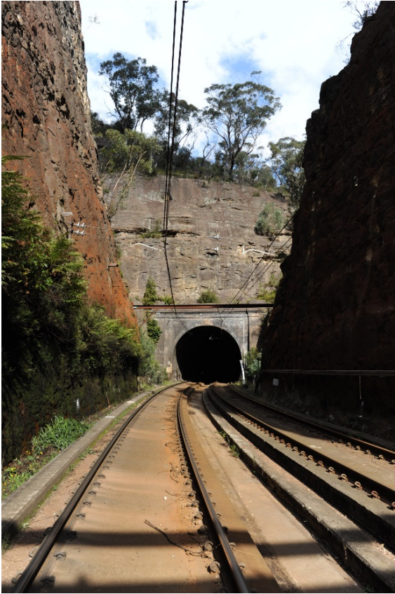
Figure 92: Lithgow end portal, Tunnel 7
