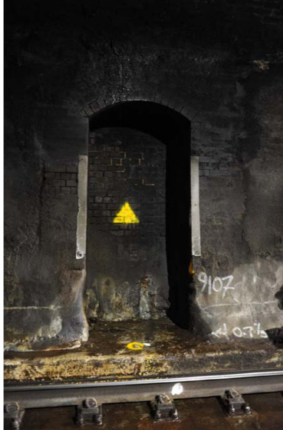
Figure 120: Brick lined 'recess' in tunnel lining, showing existing notching
