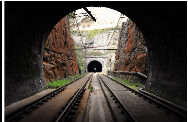
Figure 74: View from Sydney end portal of Tunnel 5 towards of Tunnel 4
