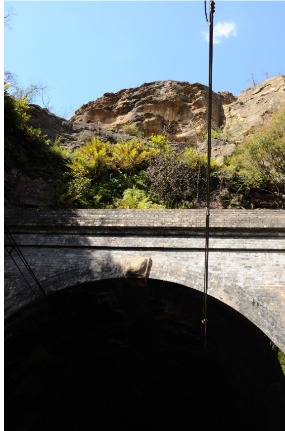
Figure 59: View of portal entrance to Tunnel 3 and sandstone cliff overhead
