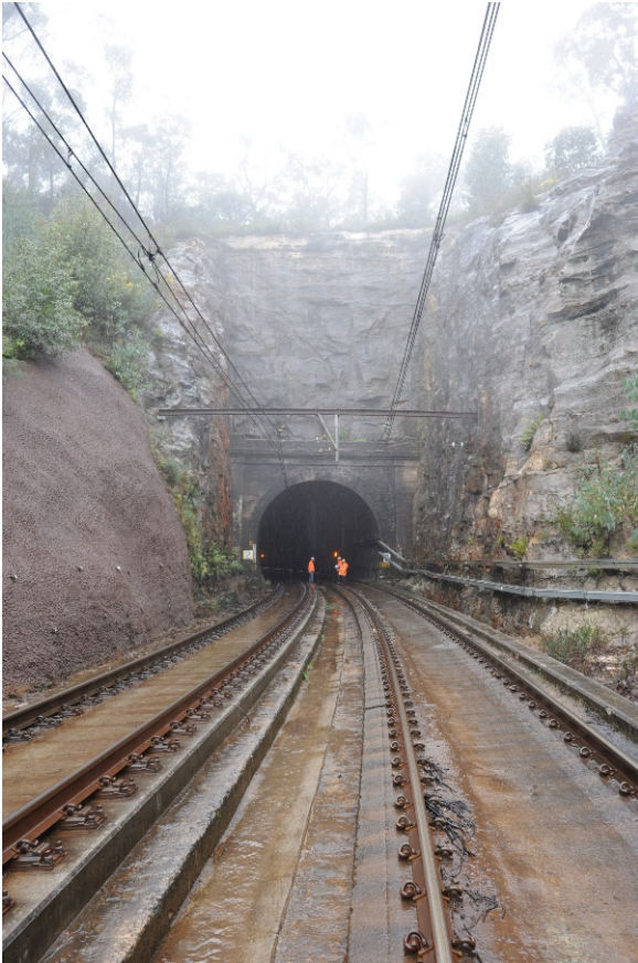
Figure 49: Lithgow end portal of Tunnel 2
