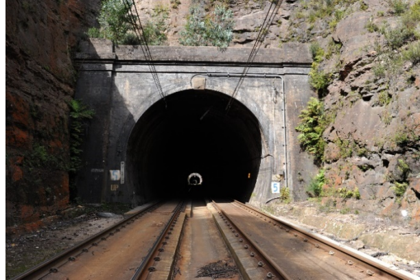
Figure 70: Lithgow end portal, Tunnel 5
