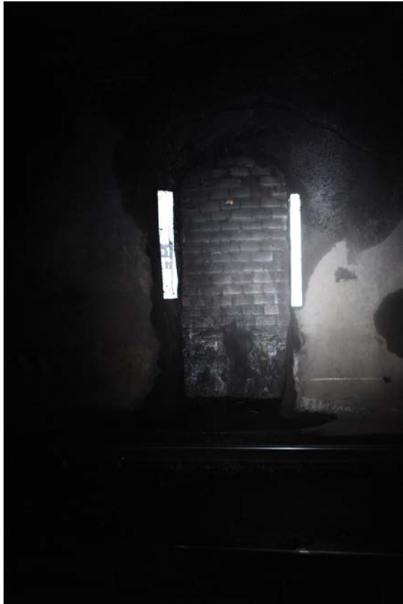
Figure 101: Brick lined 'recess' in tunnel lining
