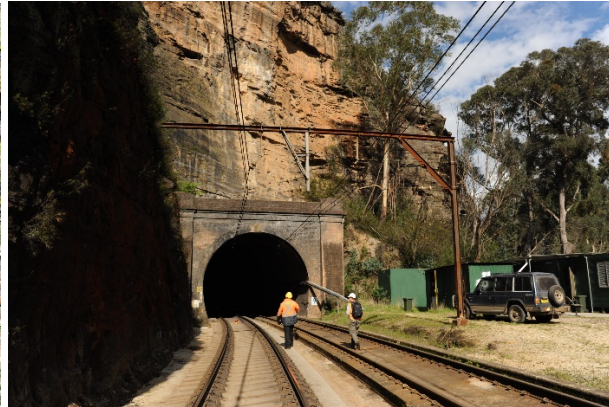
Figure 105: Lithgow end portal, Tunnel 9 showing adjacent compound area
