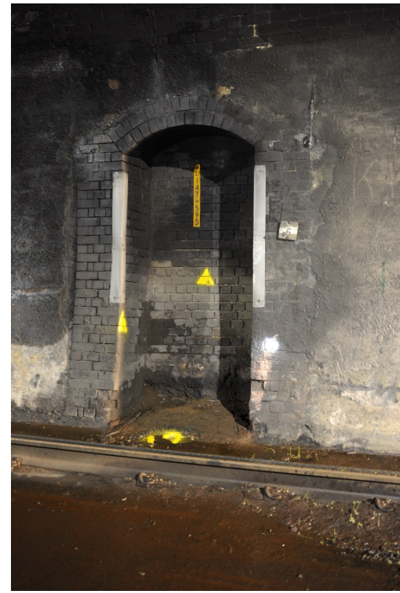
Figure 68: Brick lined 'recess' in tunnel lining
