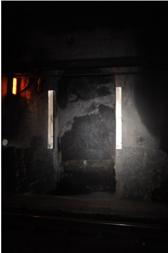
Figure 84: 'Recess' in tunnel lining
