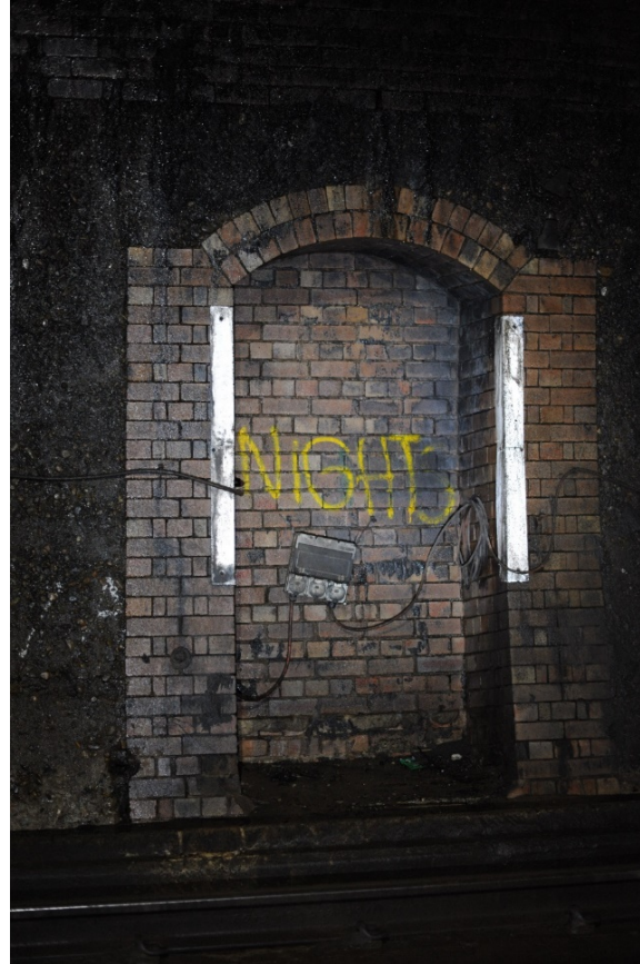
Figure 41: Brick lined 'recess' in tunnel wall
