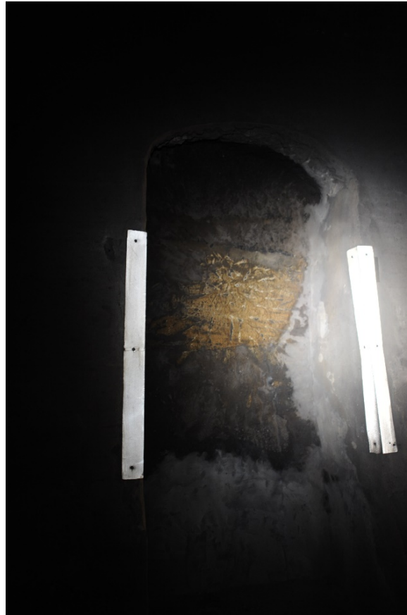
Figure 50: Recess – later addition
