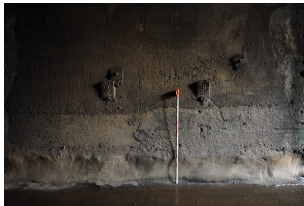
Figure 90: Detail of existing toe notching and gradient/radius/survey markers within Tunnel 7
