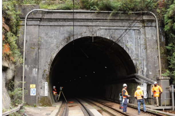
Figure 114: Lithgow end portal, Tunnel 10
