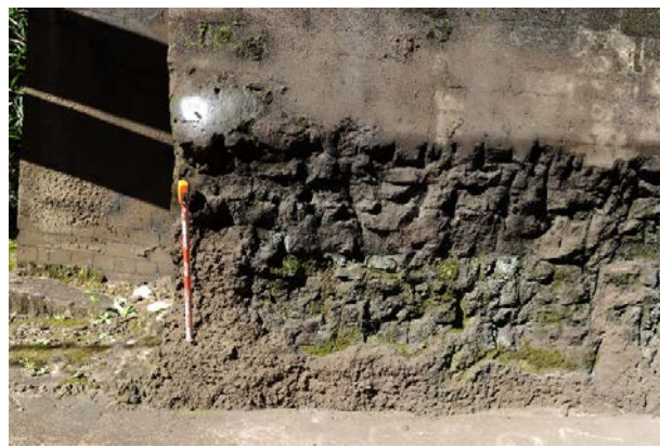
Figure 47: Detail photo of existing notching, down track Sydney end portal
