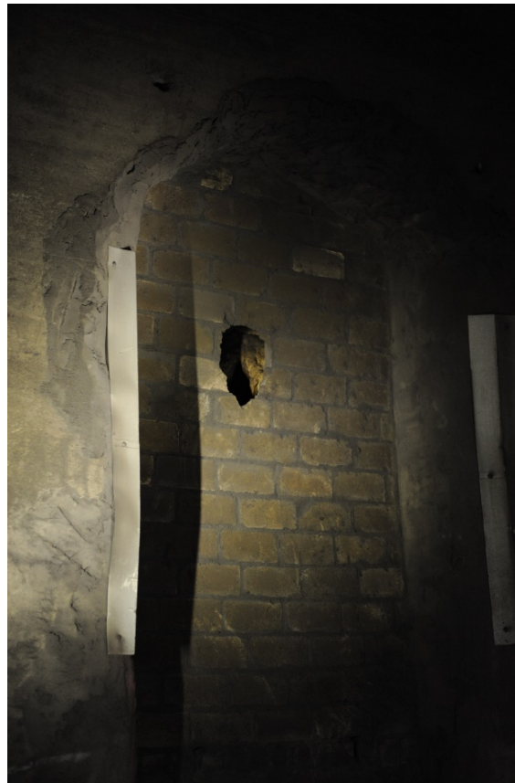
Figure 102: Brick lined 'recess' in tunnel lining
