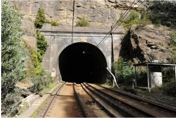
Figure 86: Lithgow end portal, Tunnel 7
