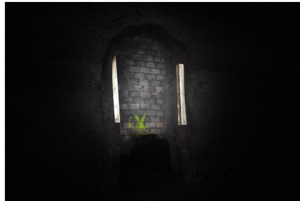
Figure 73: Brick lined 'recess' in tunnel lining
