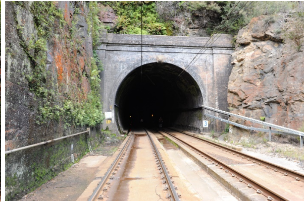
Figure 53: Lithgow end portal, Tunnel 3
