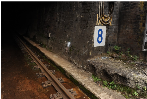
Figure 98: Detail shot of toe section of Tunnel 8 showing absence of notching, down track
