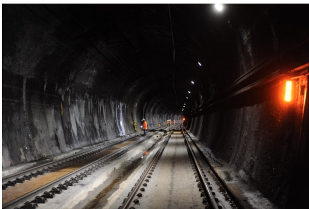
Figure 116: Internal view within Tunnel 10 showing existing lighting
