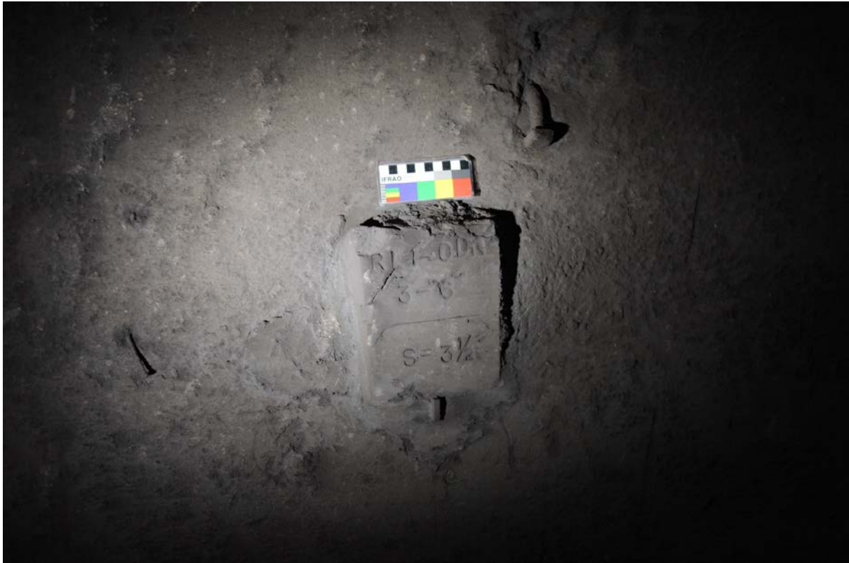
Figure 22: Example of gradient/ radius/ survey marker, Tunnel 10 down track
