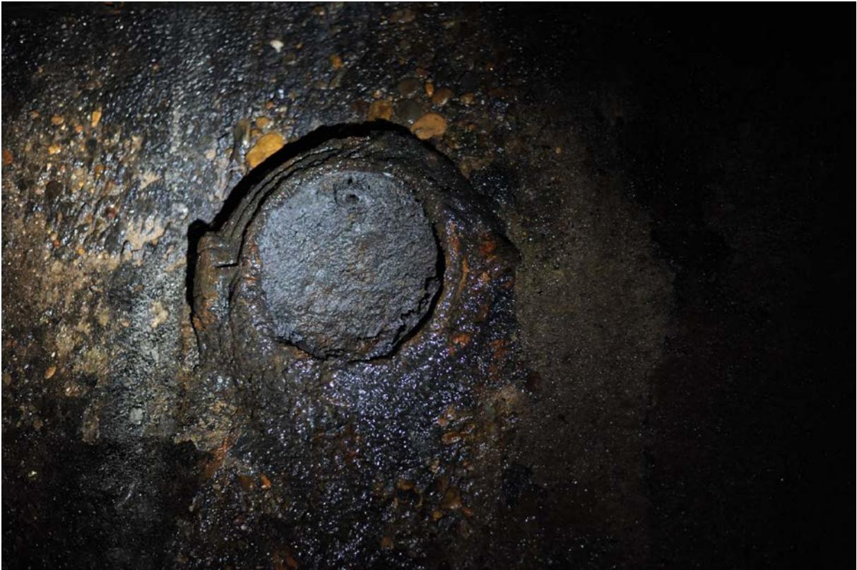
Figure 20: Example of former light fitting, Tunnel 1 down track
