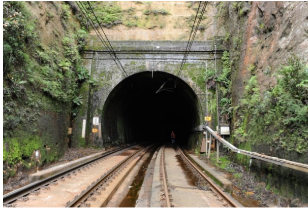
Figure 35: Lithgow end portal, Tunnel 1
