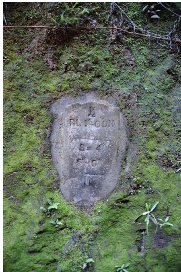
Figure 23: Example of gradient/ radius/ survey marker, down track cutting face adjacent Tunnel 1 Lithgow end portal
