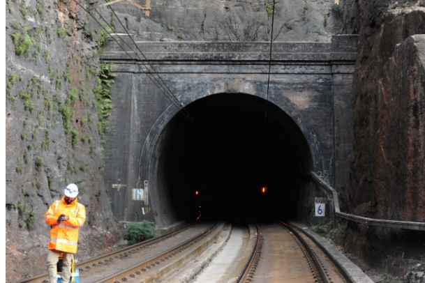
Figure 79: Lithgow end portal, Tunnel 6
