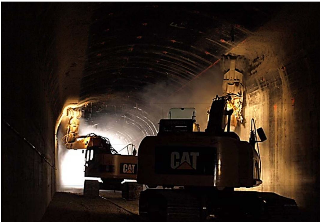
Figure 123: Example of excavator machinery with cutter head attachment
