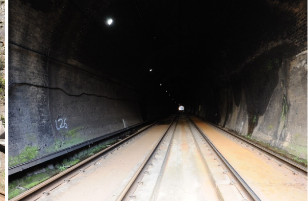
Figure 62: View of Tunnel 4 interior showing tunnel lining
