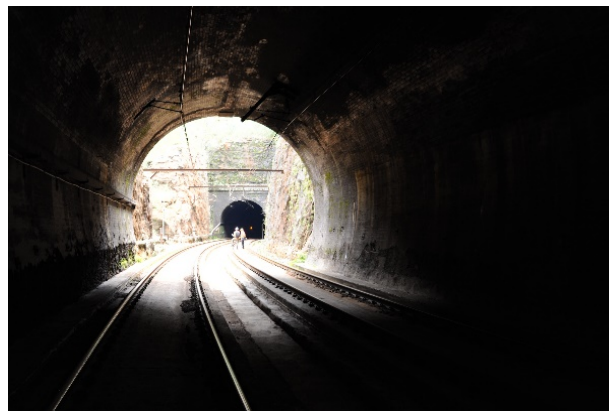
Figure 82: Internal view of Tunnel 6 towards Tunnel 7
