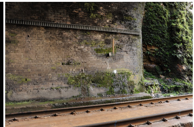
Figure 57: up track tunnel lining, Tunnel 3
