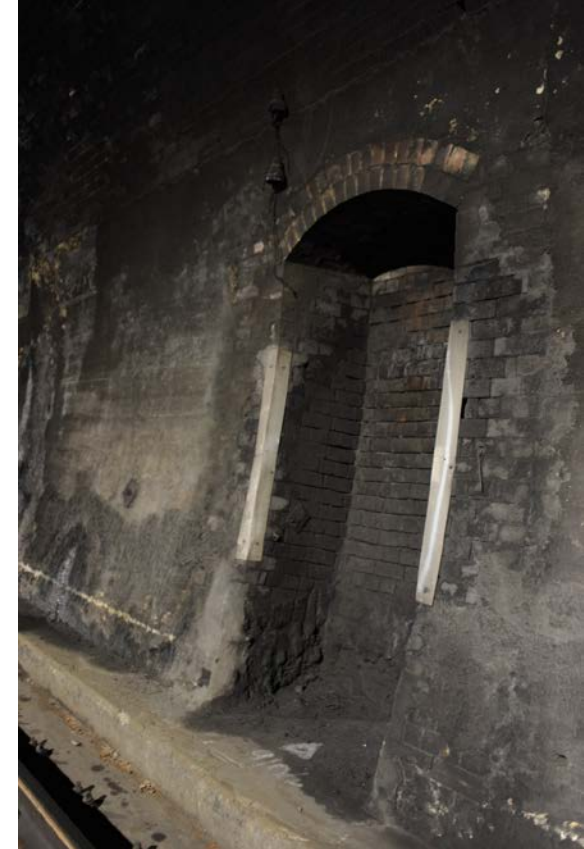
Figure 121: Brick lined 'recess' in tunnel lining
