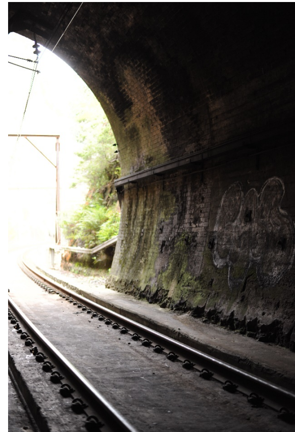
Figure 103: Detail shot of brick lined toe section of Tunnel 8, down track
