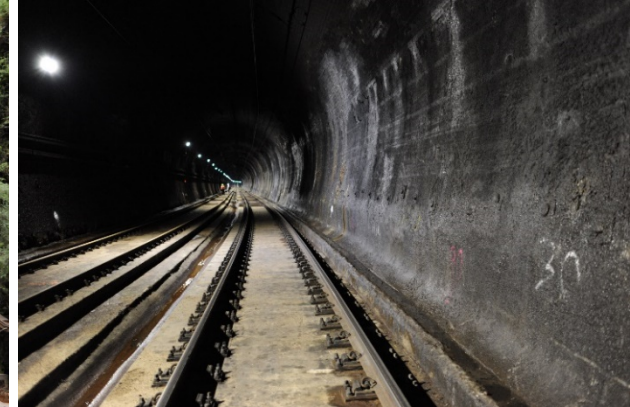
Figure 115: Internal view within Tunnel 10 showing rock bolts and existing notching
