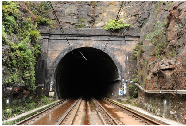
Figure 96: Lithgow end portal, Tunnel 8
