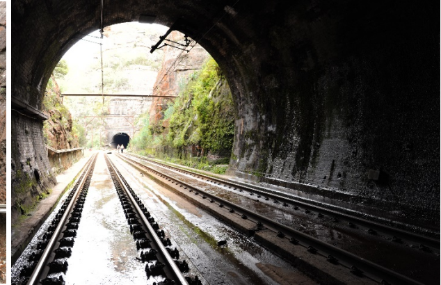
Figure 97: Internal view within Tunnel 8 towards Sydney end portal of Tunnel 9
