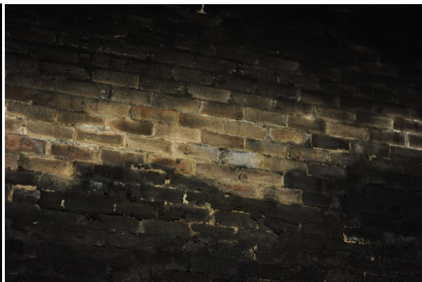
Figure 64: Detail shot of brick vault within Tunnel 4
