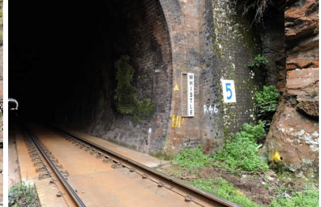
Figure 71: Detail of brick lining, up track
