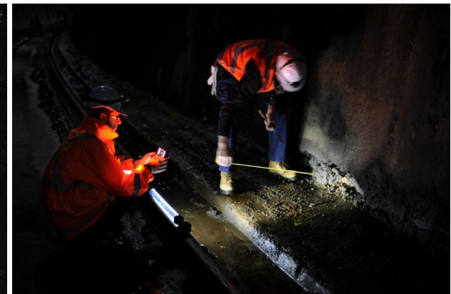
Figure 39: Tunnel Engineers documenting condition of original concrete fabric
