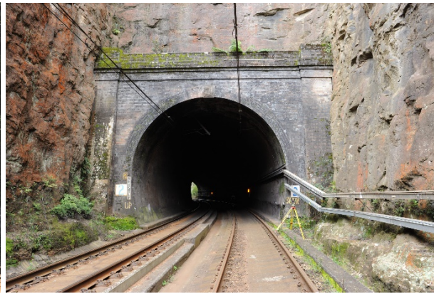
Figure 44: Lithgow end portal, Tunnel 2
