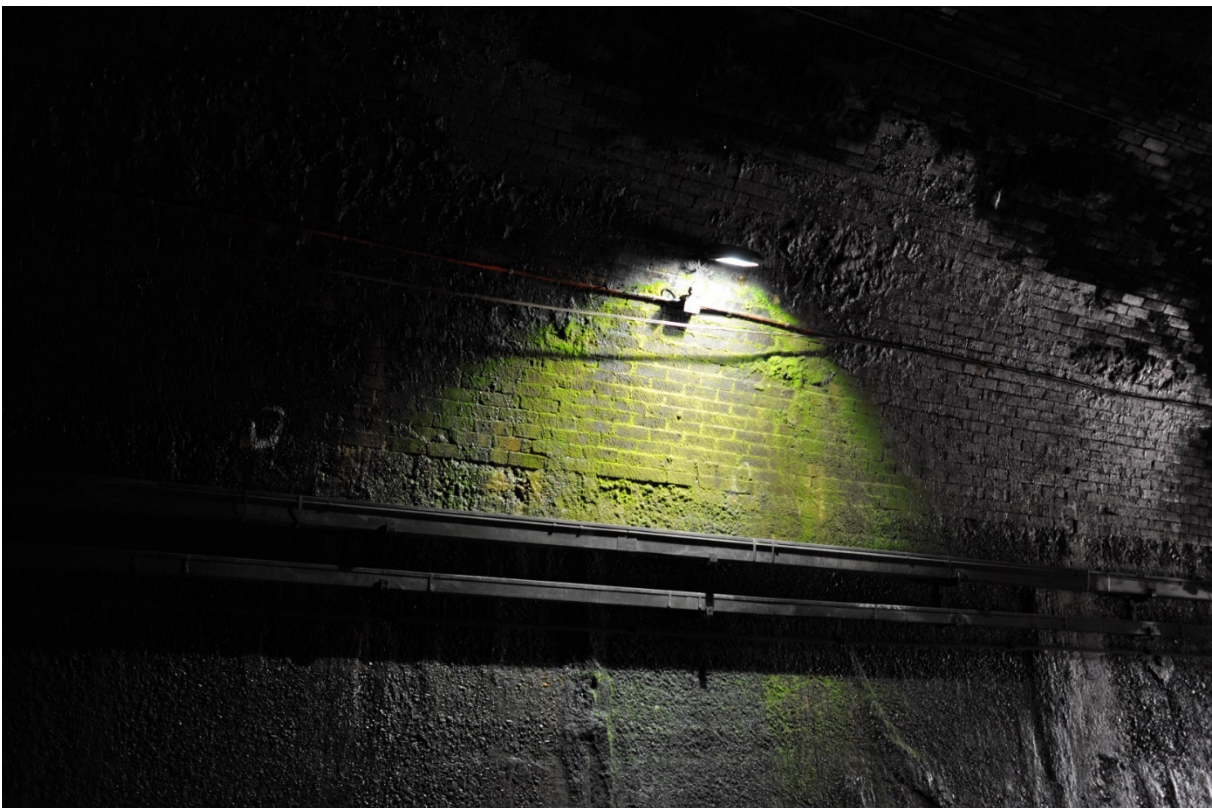
Figure 17: Example of stretcher bond within tunnel lining, this example from Tunnel 1
