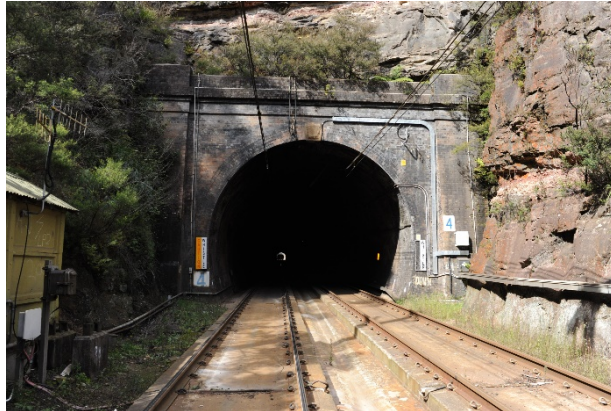
Figure 61: Lithgow end portal, Tunnel 4
