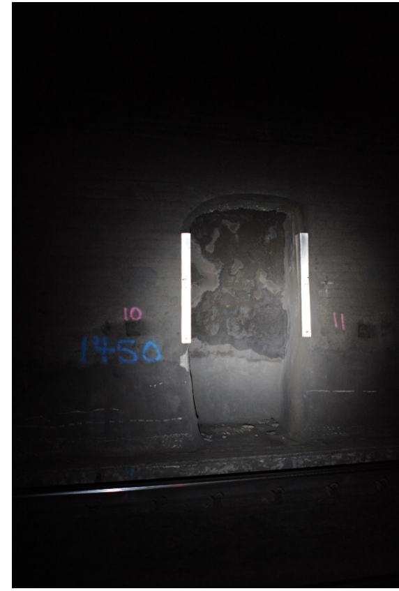
Figure 94: 'Recess' in tunnel lining
