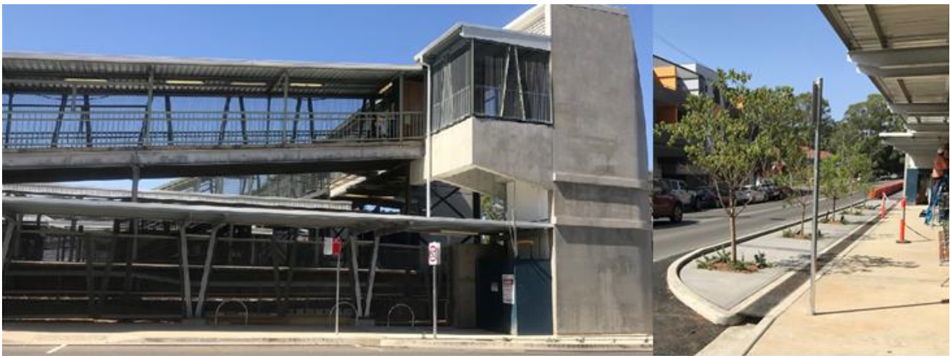
Landscaping and canopies around lift landing on Wentworth Avenue and Portico Parade
