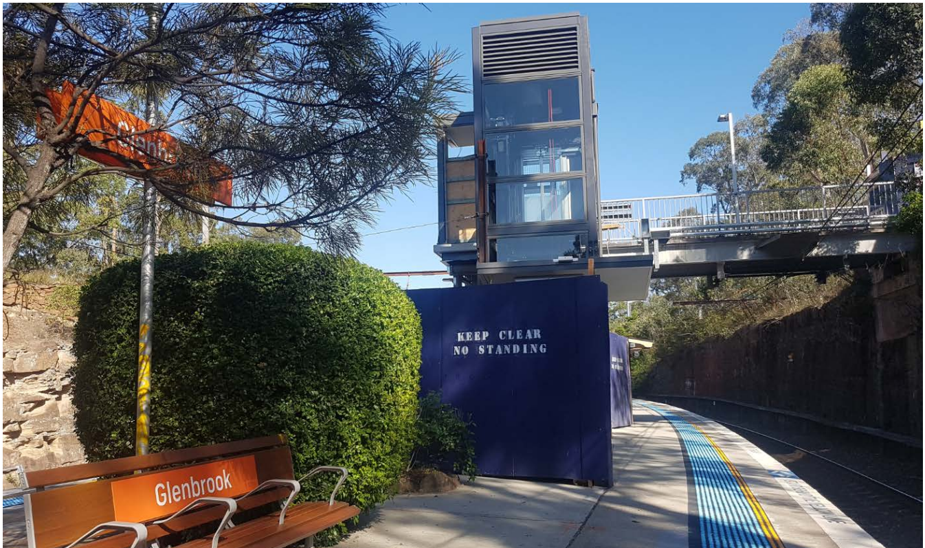
Photo of new lift shaft at Glenbrook Station
