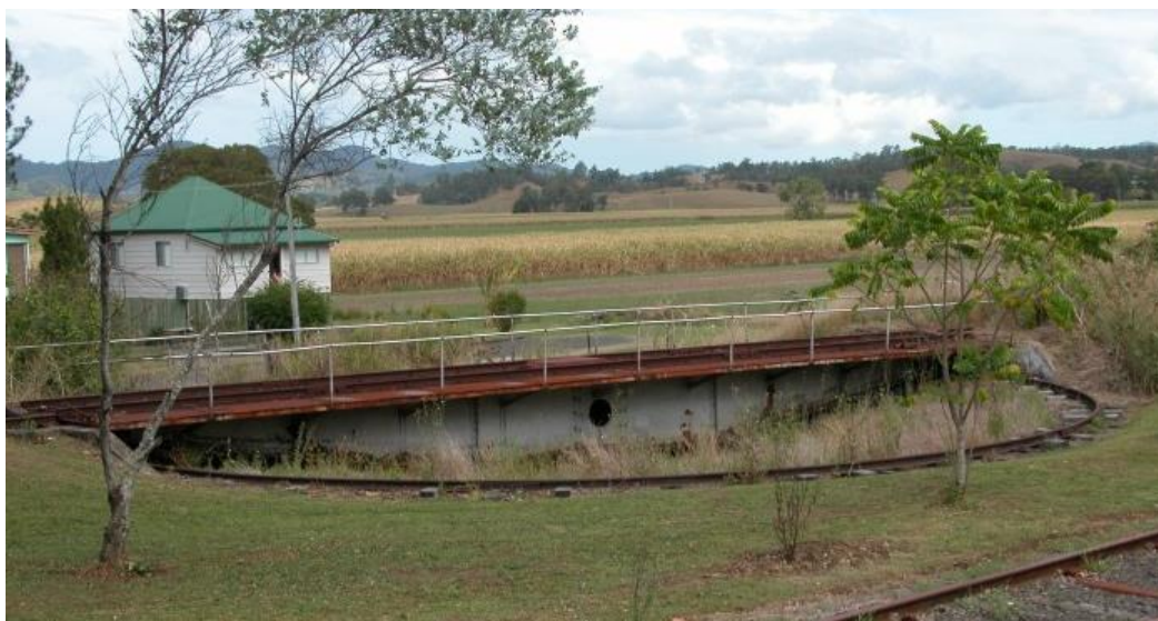
Figure 23. Murwillumbah's 60ft railway turntable circa 2005. Note the lowered side walls and concrete wings below the railway track at either end. (Source: RailNet).
