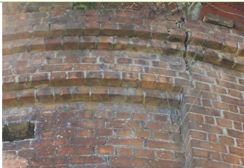
Figure 51. This brickwork crack is moving vertically downwards and is apparent on the inside of the brickwork as well.
