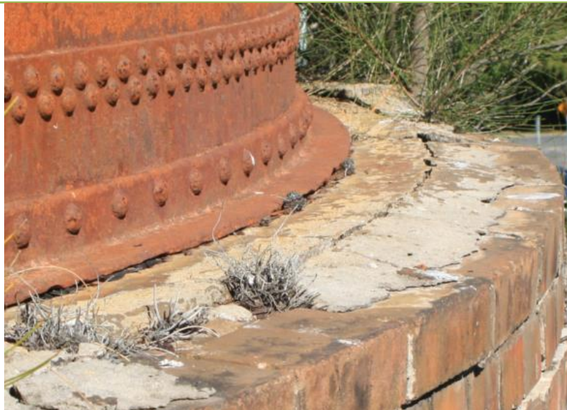
Figure 47. The lower flange attached to the tank and the rendered coping on the brickwork were designed to shed stormwater but both are in poor condition.
