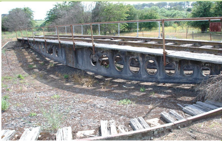
Figure 55. The turntable at Crookwell, NSW demonstrates one of the simplest arrangements (Flickr – J Webb)
