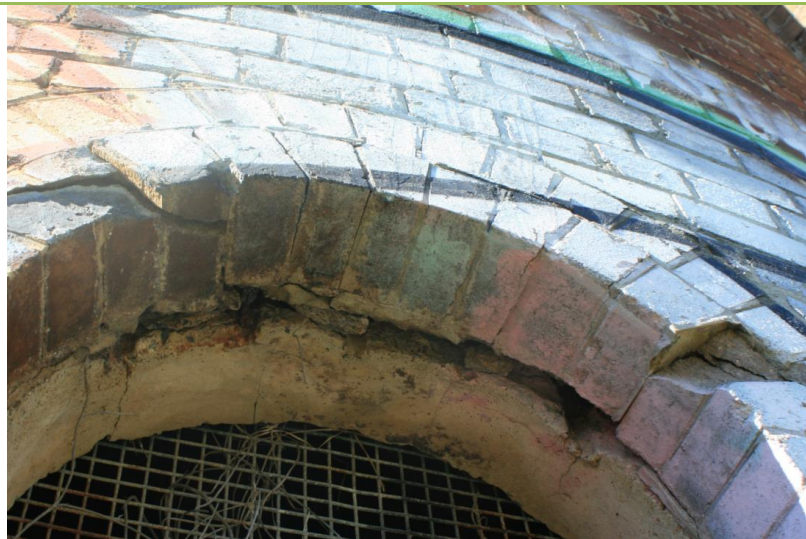
Figure 50. The arch brickwork of the western window has moved and one brick has been crushed.
