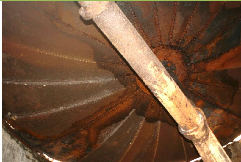
Figure 43. The underside of the water tank and outlet piping viewed from within the brick tower. The tank floor appears to be relatively sound.
