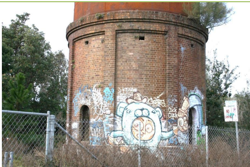
Figure 42. The brick tower is generally in good condition, except where affected by vegetation and metal corrosion around the top.
