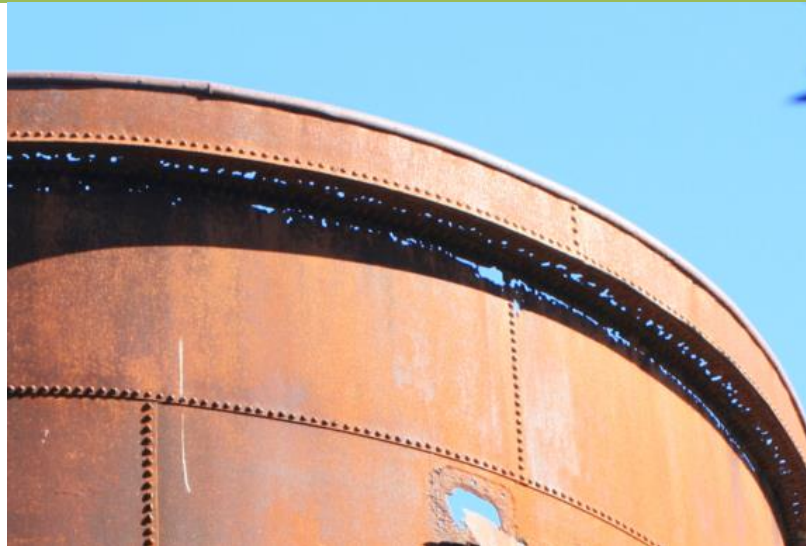
Figure 49. The corrosion of the upper horizontal tank lip appears more advanced than corrosion of the vertical surfaces.
