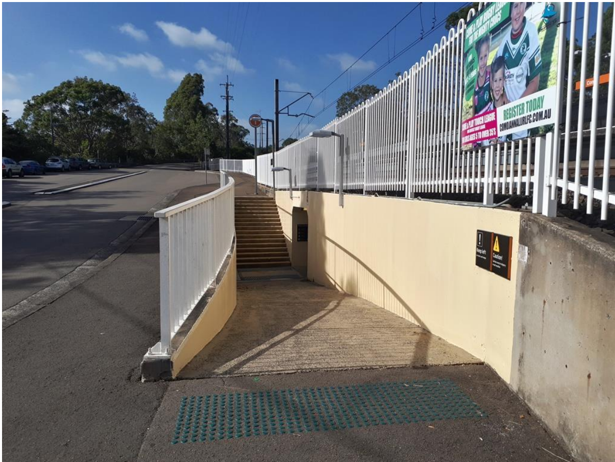
Figure 6 Como Station eastern pedestrian access point looking south from Railway Road
