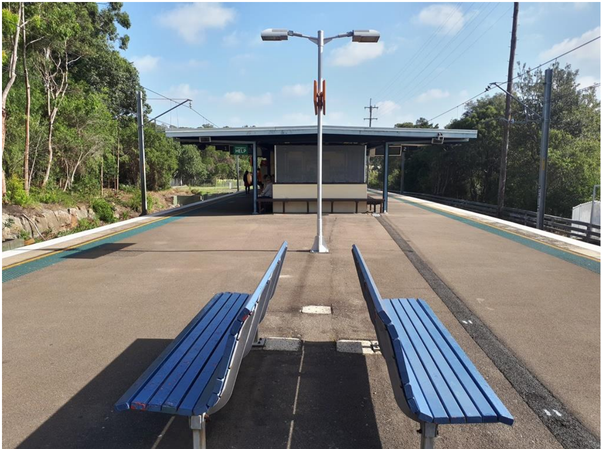
Figure 5 Como Station platform looking south, showing Platform 1 and Platform 2
