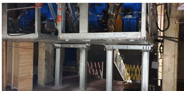
Images: Escalator 3 & 4 construction progress
