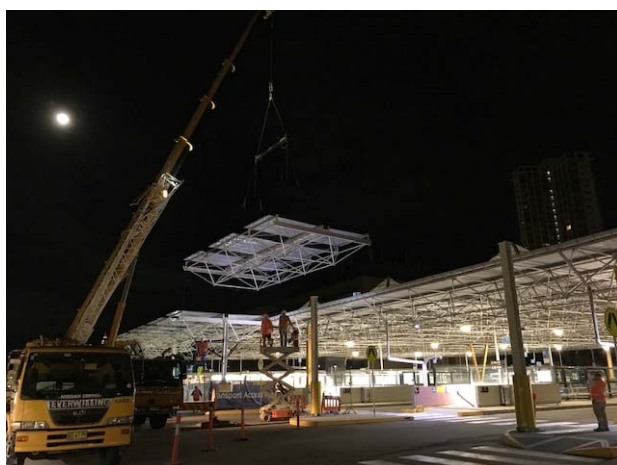
Images: Bus Canopy craneage installation
