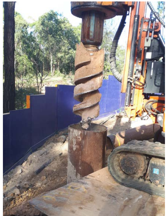
Piling work for new walkway from Burfitt Parade to footbridge
