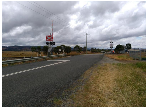
Hoskinstown Road, Bungendore (After)
