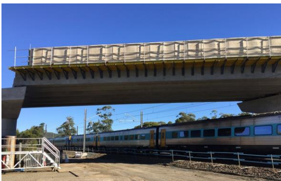
Access bridge girders in place over the rail line (looking south)
