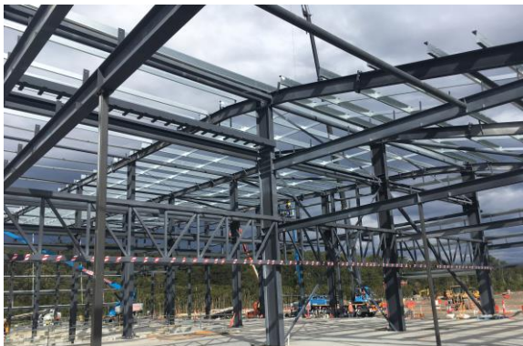
Structural steel for the main building of the maintenance facility
