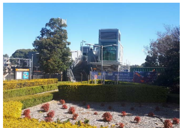
Photo of the lift shaft at North Strathfield Station
