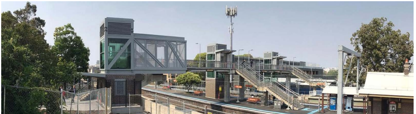
Panoramic view showing the three new lifts at North Strathfield Station
