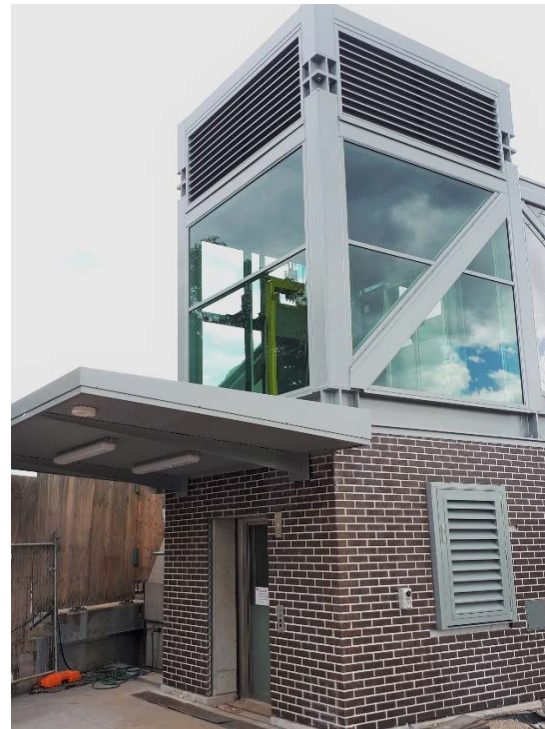
Photo of the lift at North Strathfield Station
