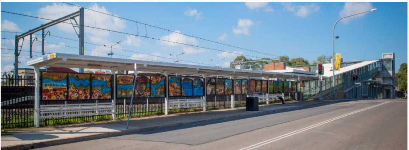
Completed works at Toongabbie station
