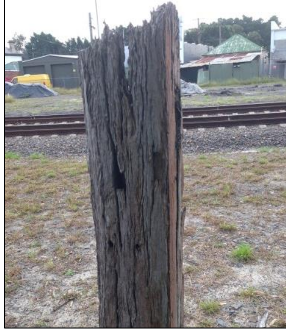
PICTURE 4 – CLOSE DETAIL OF TIMBER RELIC
