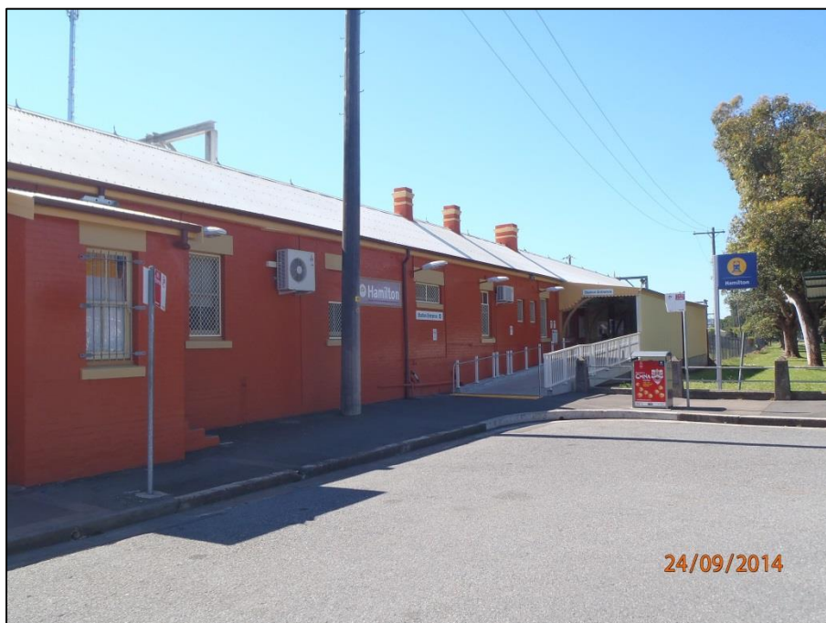
FIGURE 4 – SOUTHERN STATION ENTRANCE – PLATFORM 1
