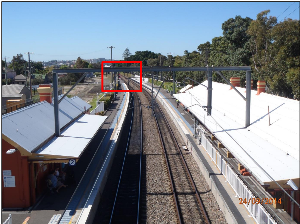
FIGURE 2 – VIEW OF HAMILTON RAILWAY STATION GROUP SHOWING THE LOCATION OF THE PROPOSED EXTENSION TO PLATFORM 2 (RED BOUNDARY)
