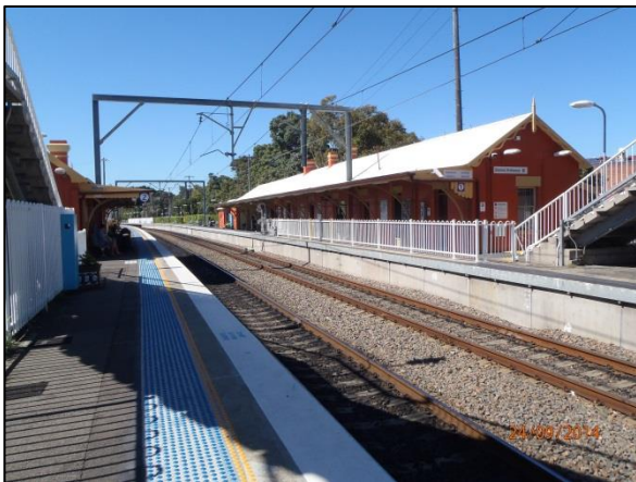
PICTURE 1 – VIEW OF STATION PLATFORMS FROM PLATFORM 2, FACING SOUTHEAST
