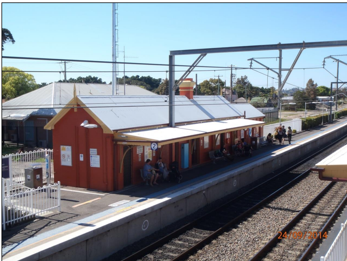
FIGURE 5 – VIEW OF PLATFORM 2 FROM THE PEDESTRIAN FOOTBRIDGE, FACING NORTHEAST
