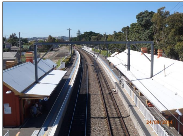
PICTURE 2 – VIEW OF PLATFORMS FROM FOOTBRIDGE, FACING SOUTHEAST
