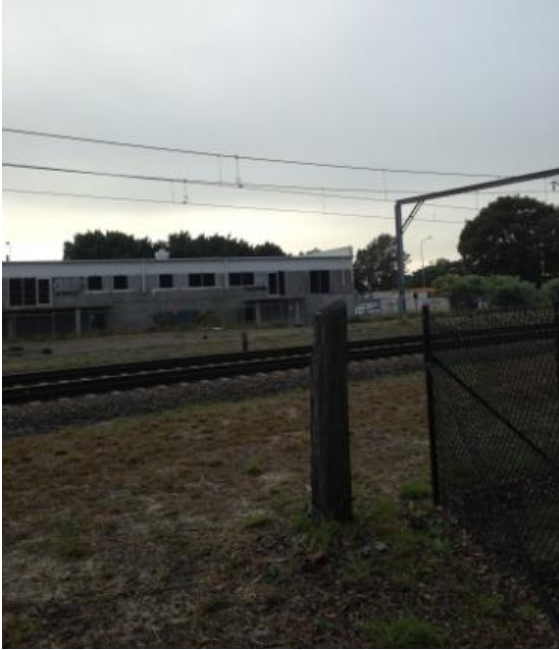
PICTURE 3 – VIEW OF TIMBER RELIC IN RELATION TO ITS SURROUNDING CONTEXT
