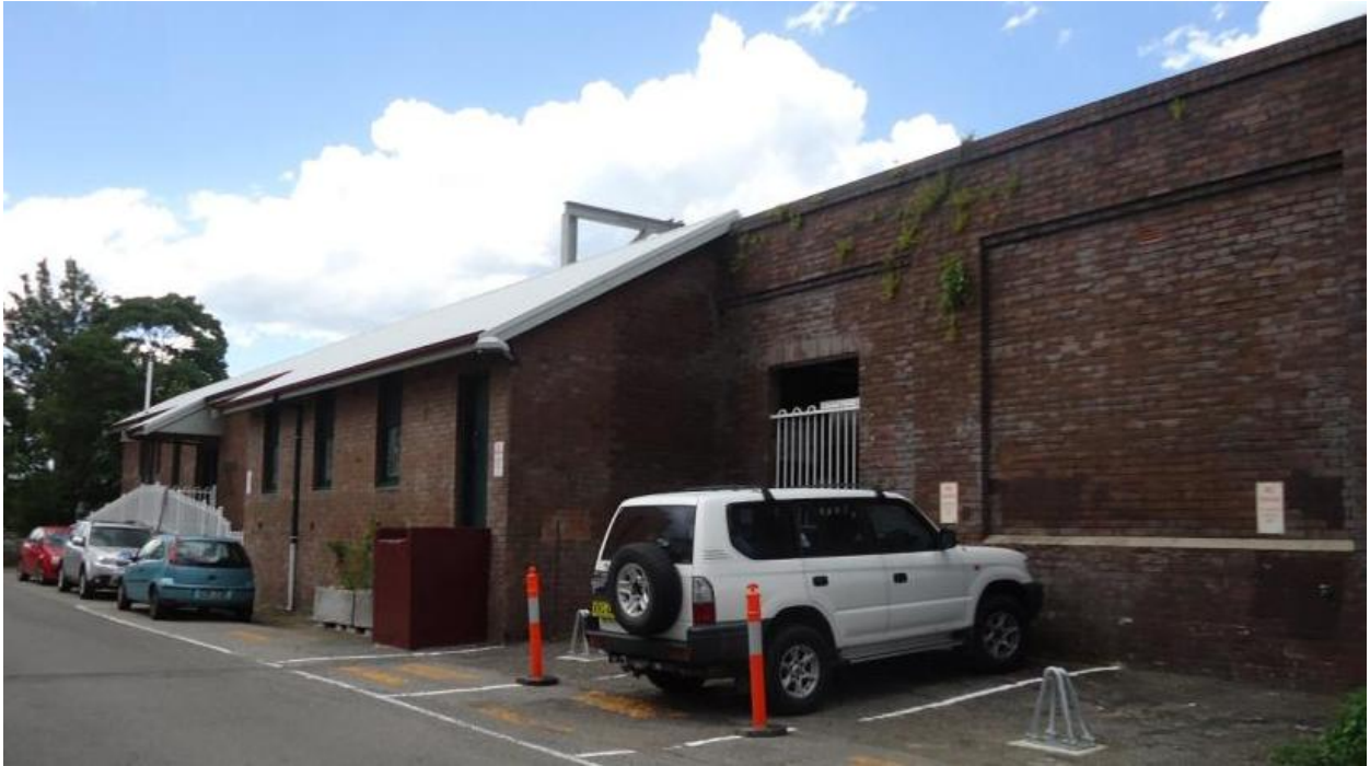
FIGURE 17 – SOUTHERN ELEVATION OF STATION AS VIEWED FROM BERESFORD STREET
