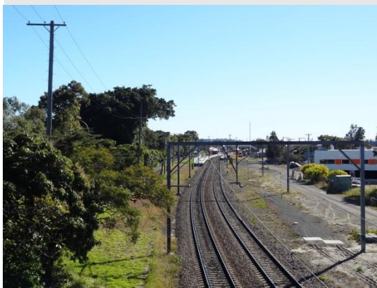
Photo 5 VP4 Maitland Road overbridge - view to the north-west along the rail corridor from Maitland Road overbridge towards Beaumont Street.
