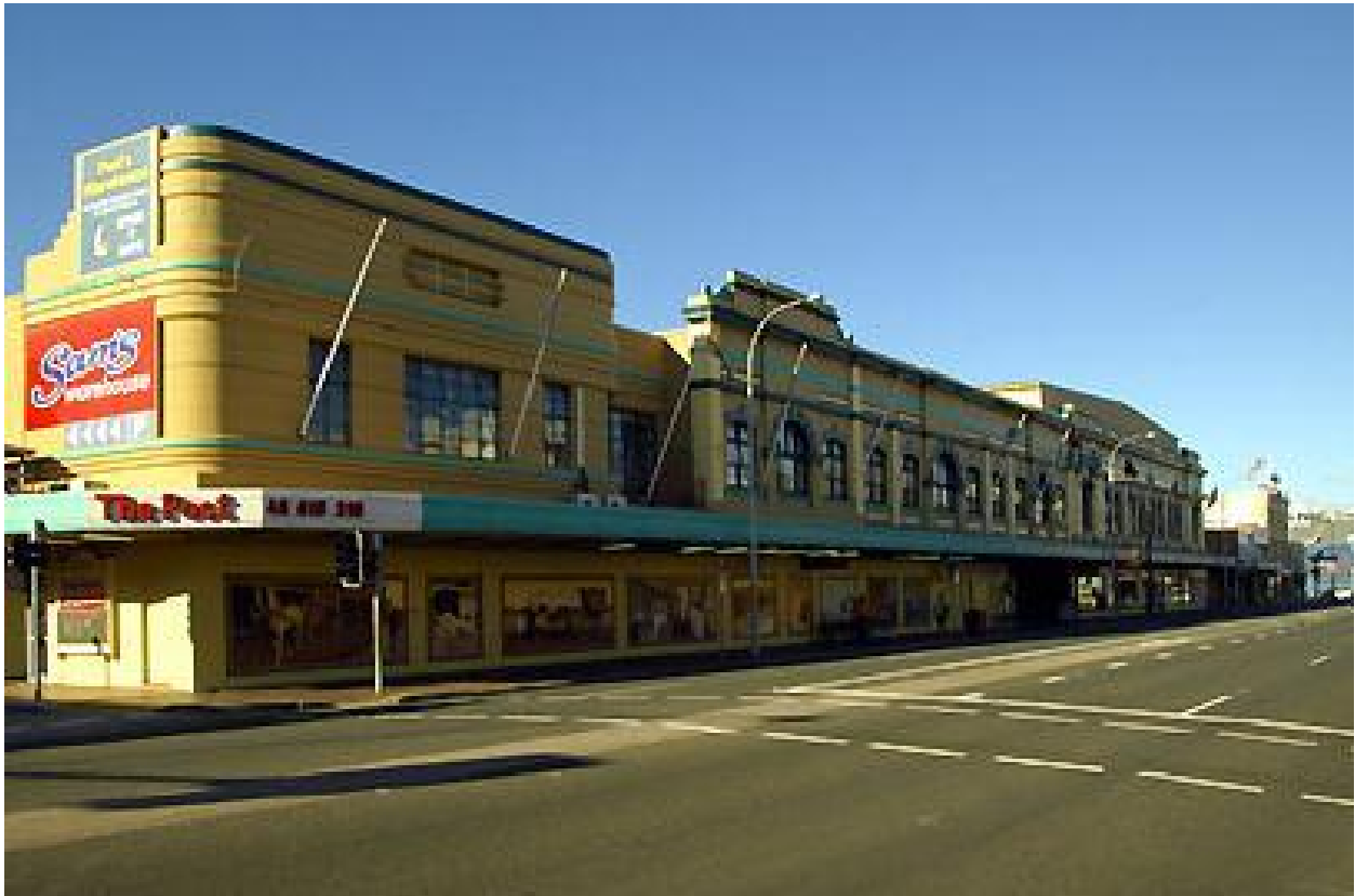
FIGURE 12 – VIEW OF FORMER NEWCASTLE COOPERATIVE STORE FAÇADE ON HUNTER STREET
