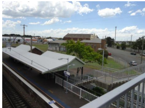
PICTURE 6 – VIEW OF PLATFORM 2 FROM FOOTBRIDGE
