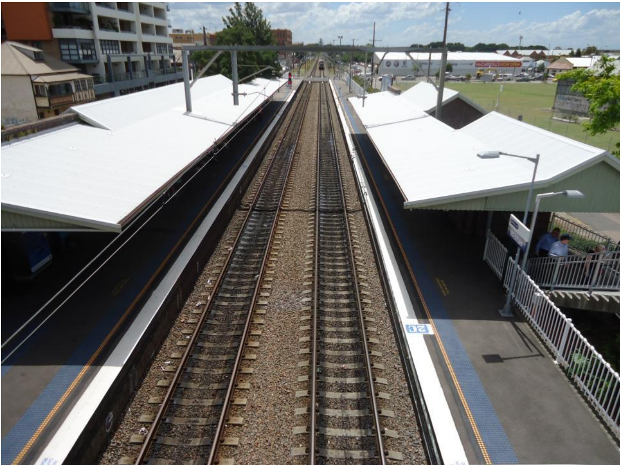
FIGURE 16 – VIEW OF WICKHAM STATION, PLATFORMS 1 AND 2, LOOKING TOWARD STEWART AVENUE
