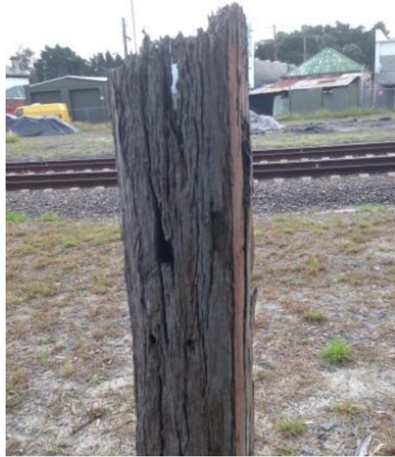
PICTURE 4 – CLOSE DETAIL OF TIMBER RELIC
