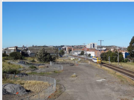
Photo 6 VP4 Maitland Road overbridge - view to the south-east along the rail corridor from Maitland Road overbridge towards Stewart Avenue.
