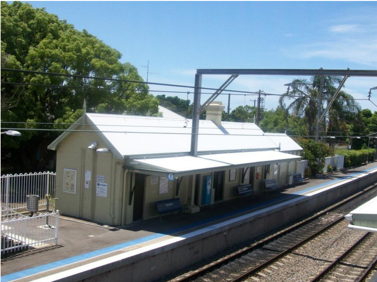
FIGURE 7 – VIEW OF PLATFORM 2 FROM THE PEDESTRIAN FOOTBRIDGE
