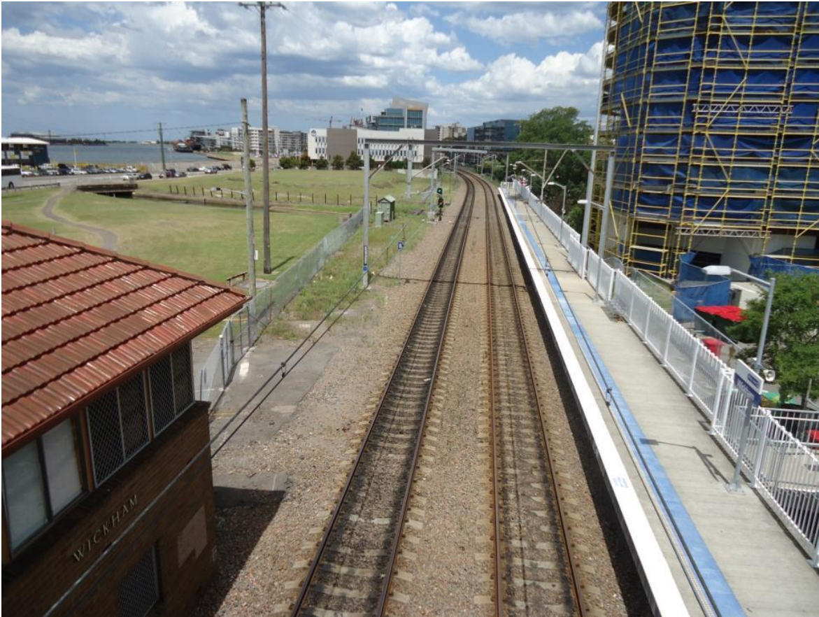
FIGURE 19 – VIEW SOUTHEAST SHOWING EXTENDED PLATFORM
