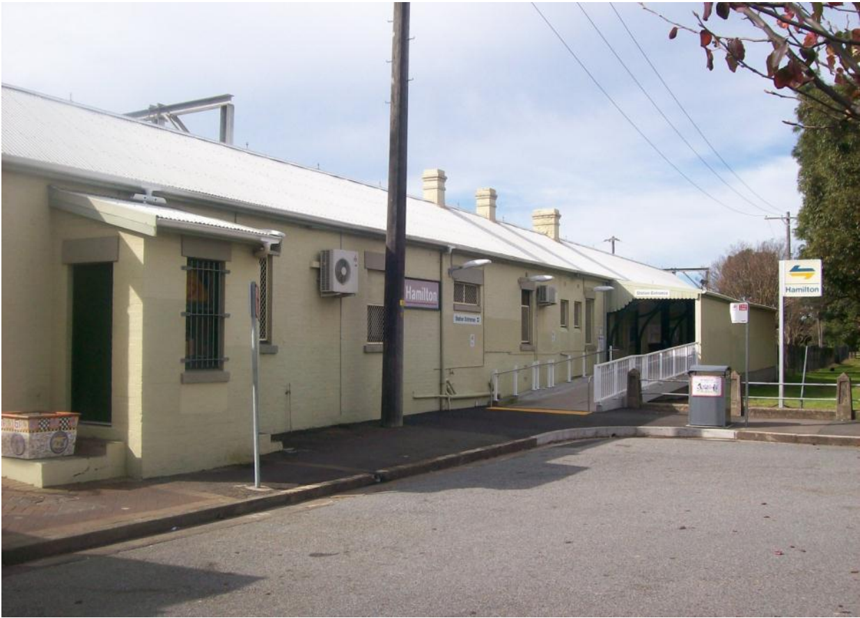
FIGURE 6 – SOUTHERN STATION ENTRANCE - PLATFORM 1
