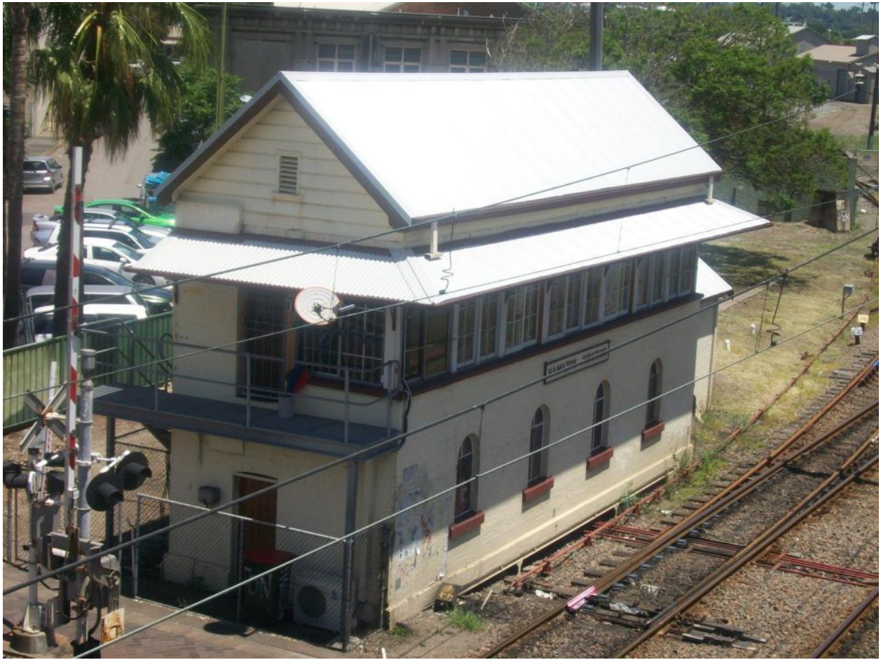
FIGURE 9 – HAMILTON JUNCTION SIGNAL BOX
