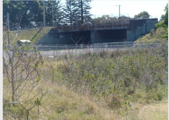
Photo 8 View south-west from Wickham Park to the Maitland Road overpass.
