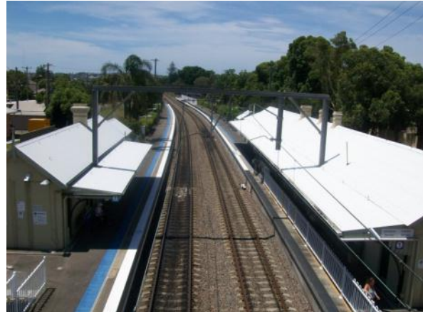
PICTURE 2 – VIEW OF PLATFORMS FROM FOOTBRIDGE
