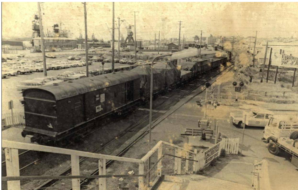
FIGURE 2 – 1970S PHOTOGRAPH OF HAMILTON STATION
