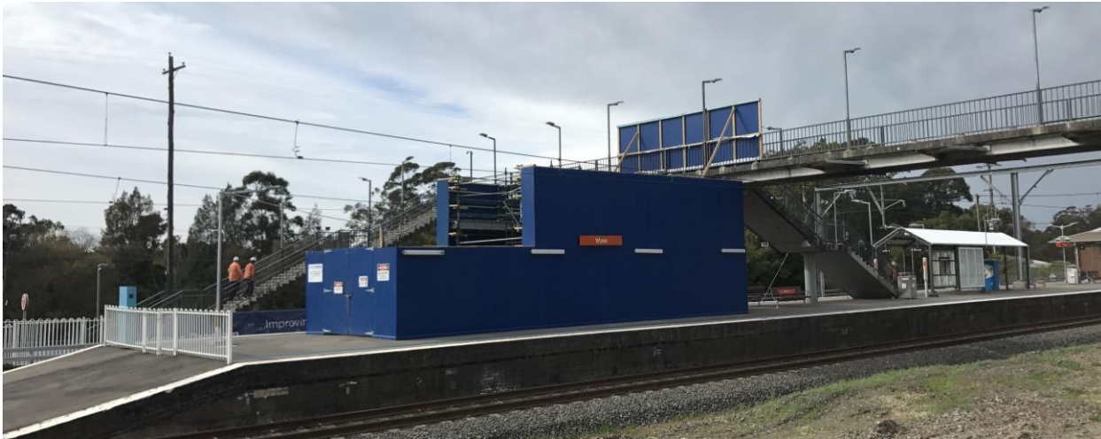
Image: Work progressing on the platform lift shaft, August 2019.
