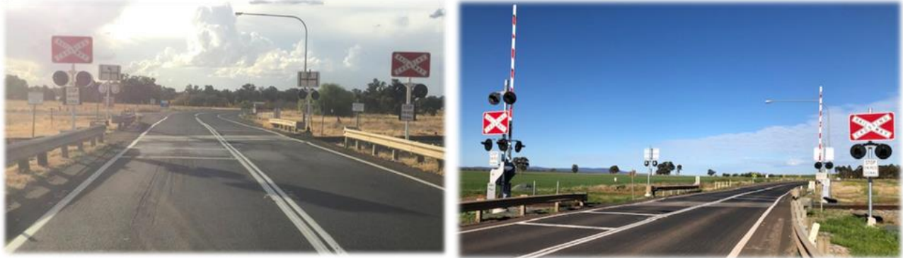
Figure 7: Newell Highway Tichborne (before and after)
