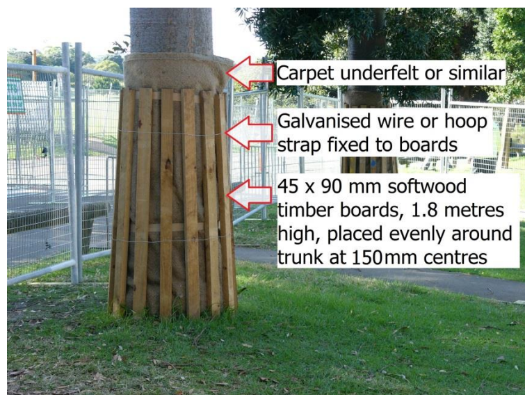
Figure 3 – Detail of Trunk Protection
