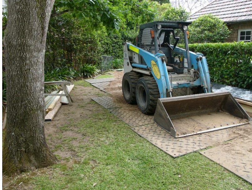
Figure 4 – Showing typical detail for truck mats.
