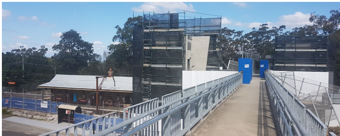
Image: Faulconbridge Station, view from footbridge looking south towards new lifts.
